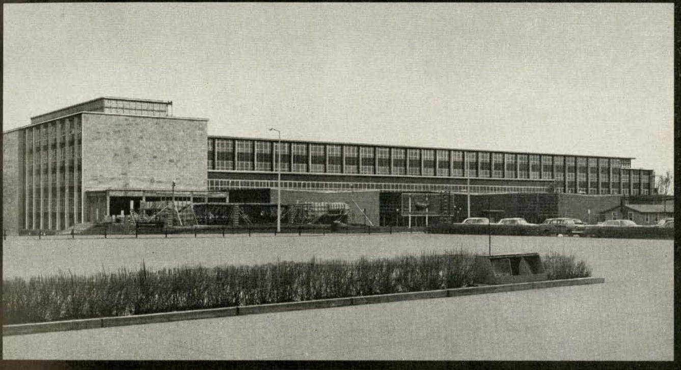
Upper left, Amqui Hospital; upper right, Bellevue Convent; lower, Applied Sciences Building, Laval University
