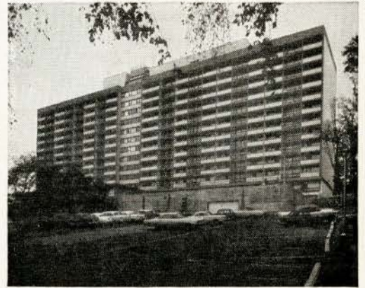
CHAMPLAIN TOWERS—Architect: Bemis, Murray and Associates General Contractor: R. Campeau
