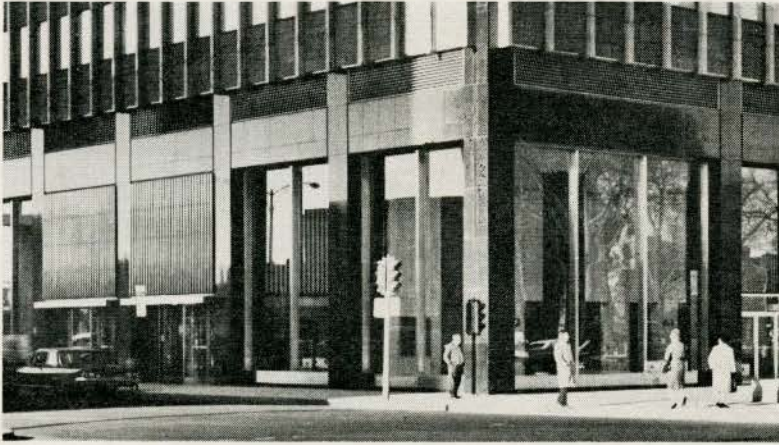
Granite facing to columns, spandrels, and the building corners to the roof level
