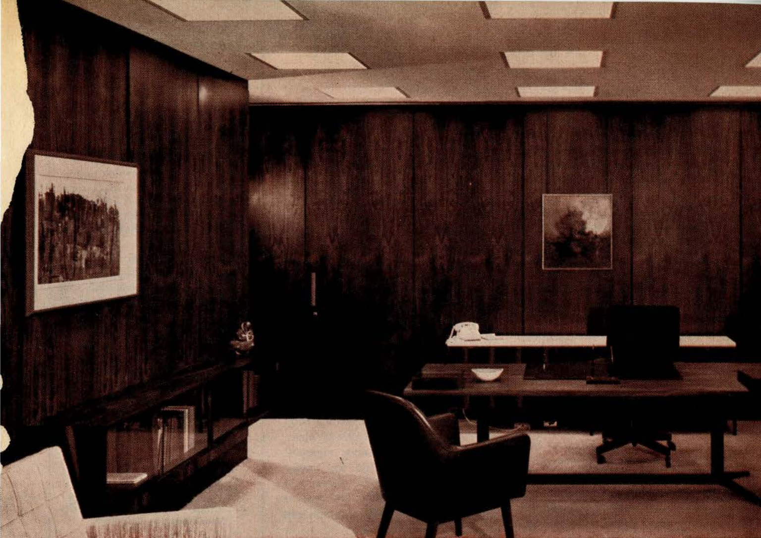
Office of the general manager, Canadian Imperial Bank of Commerce, panelled in fire-retardant, architectural, sequence-numbered Rosewood.
