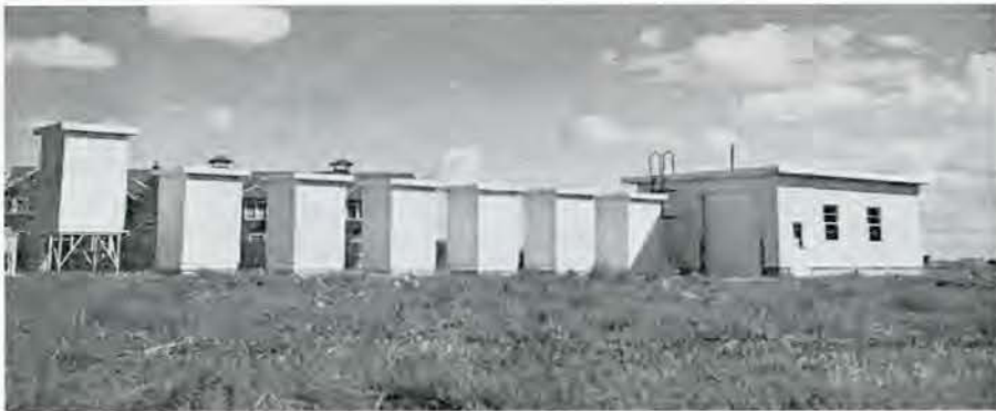
Fig. 2. Outdoor test station at Saskatoon showing the service building, six wood-frame test huts constructed over a service tunnel, and a standard hut on the left.
