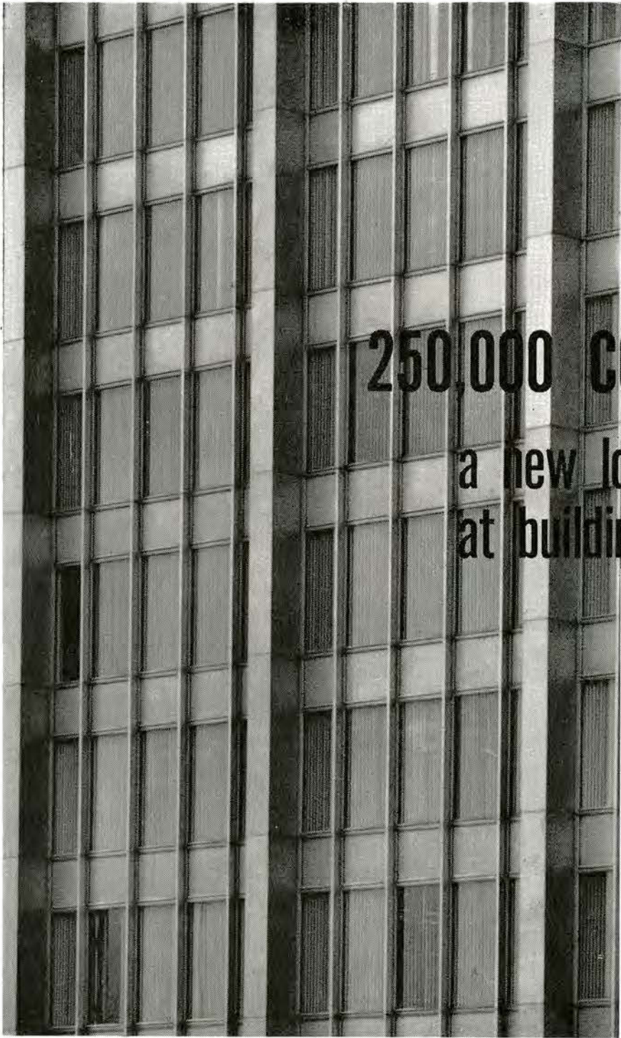
Sun Life Building, Toronto—a section of the glass and aluminum exterior showing pattern resulting from modular system of construction. Architects: John B. Parkin Associates
