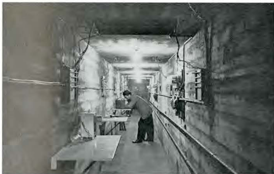
Fig. 3. View of the tunnel at Saskatoon providing access and services to the test huts above. Readings of thermocouples, power inputs and other instrumentation can be taken in the tunnel without disturbing the hut conditions.
