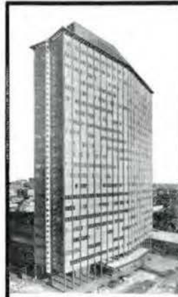
B.C. ELECTRIC BUILDING, VANCOUVER
