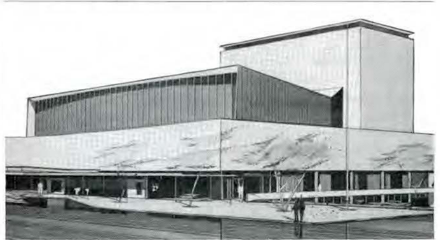
Architects: Earl C. Morgan and Page & Steele, Cons. Mech. Engineer: G. Granek & Associates
