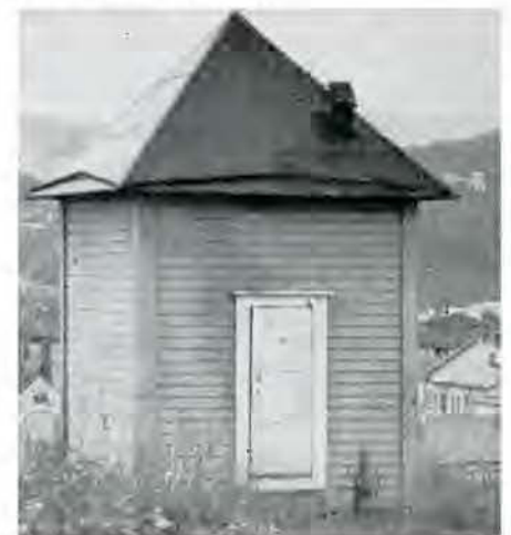
Fig. 1. One of the early test huts at Trondheim, Norway.
