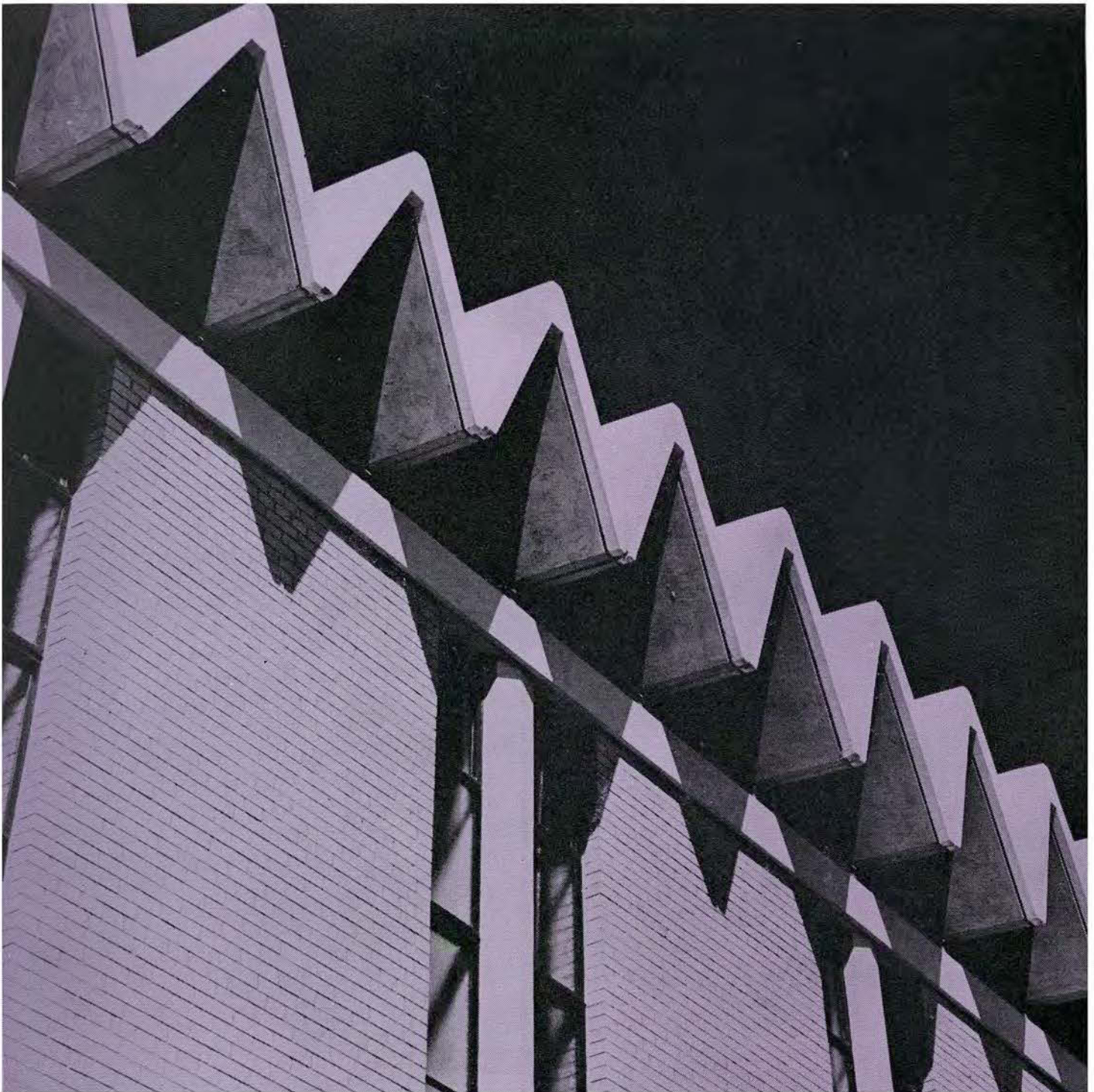
Concrete roof design by Standard Prestressed Structures Ltd. Contractor: Mollenhauer Contracting Co. Ltd. Architects & Engineers: Shore and Moffat
