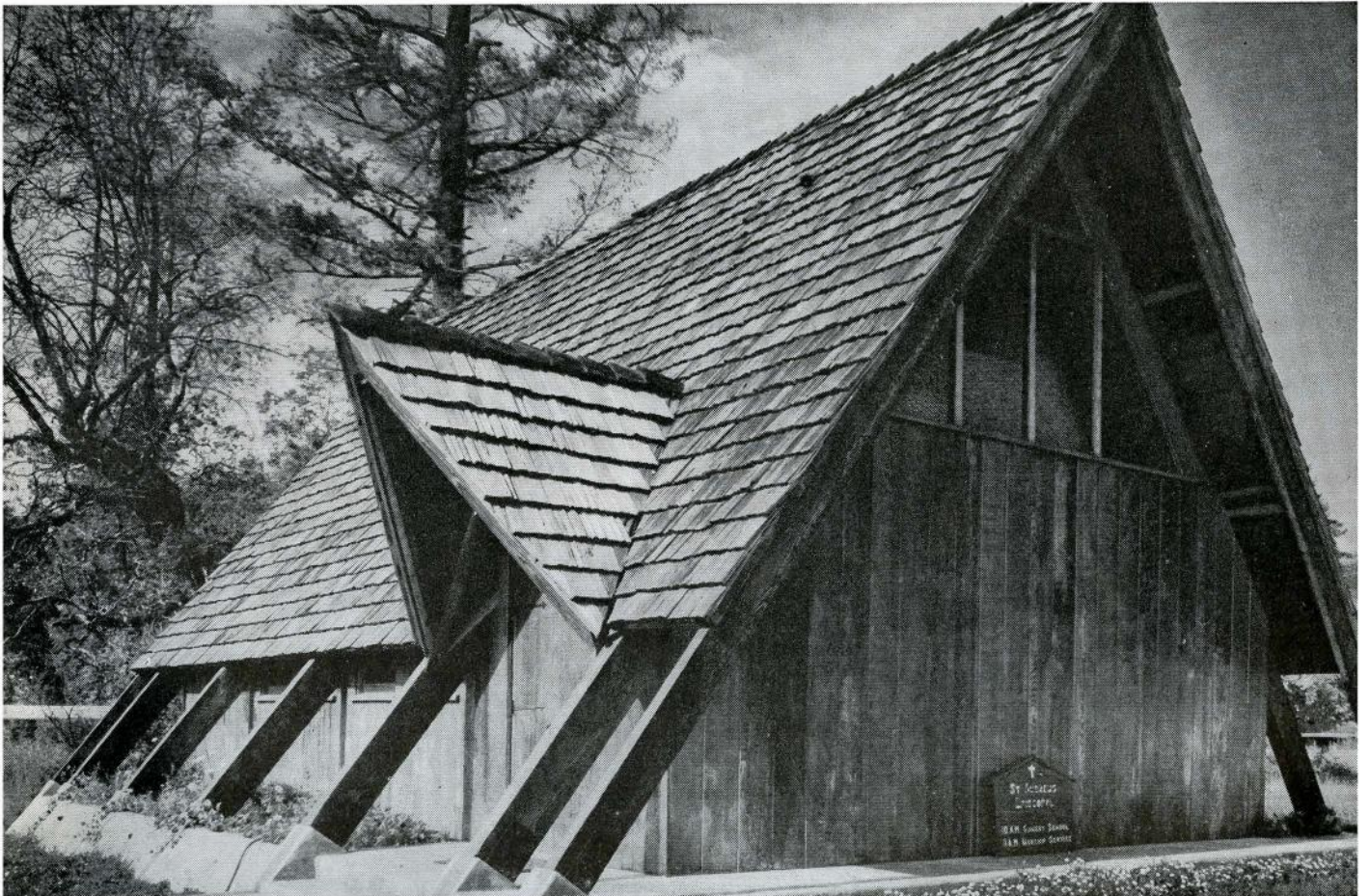
Economy in small church design uses the wood A-frame for maximum space inside. Outside, the naturally weathered handsplit shake roof, heavy A-frame supporting members, and board siding create a welcome site for worship.
