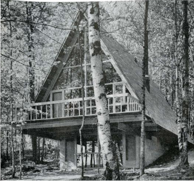
Tent-shaped A-frame vacation houses are equally at home on a coastline or in a woodland. Wood's easy portability adds to its economies and the roof-wall of wood shingles is completely weatherproof.
