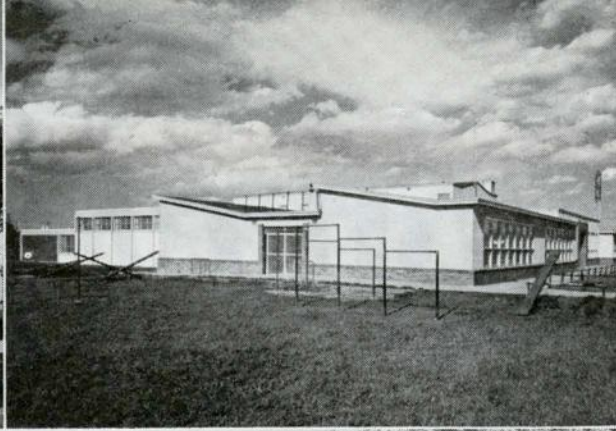
LEFT: King Edward Junior High School, Edmonton, an all concrete masonry building. Architect: John A. MacDonald . General Contractor: Universal Construction Co. Ltd.
