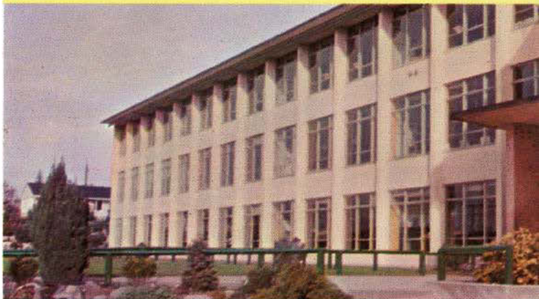
IN B.C. SIR JAMES DOUGLAS ELEMENTARY SCHOOL, VANCOUVER, B.C. Architect: Davies & McNab Architects, Vancouver, B.C. Aluminum Fabricator: Northwest Manufacturing Company Ltd.
