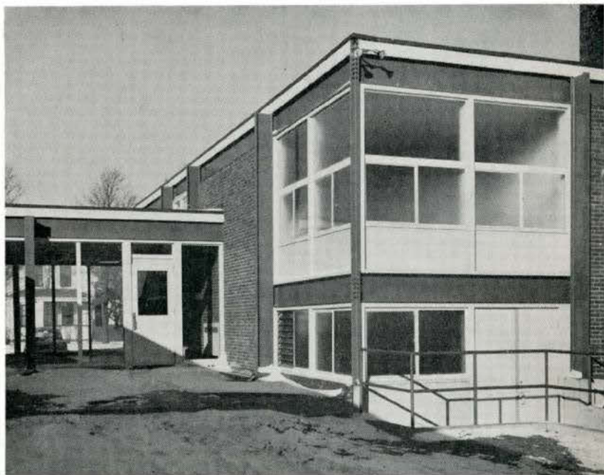
Gleaming white, baked-enamel Rusco Slim-Line Windows were contrasted with the soft grey columns, pastel colored panels and brick for lasting beauty.
