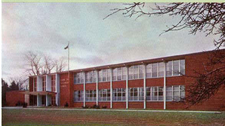
IN ONTARIO LORNE PARK SECONDARY SCHOOL, PORT CREDIT, ONT. Architect: Hanks Irwin & Pearson, Toronto, Ontario. Aluminum Fabricator: AlSCO Products of Canada, Limited
