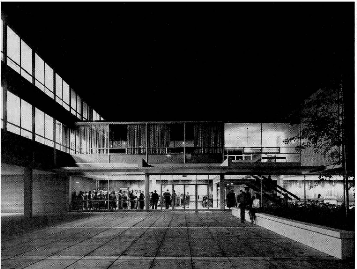
Lecture Theatre lobby
