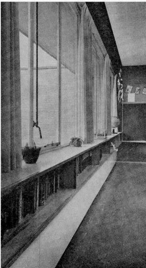
Window wall of typical classroom
