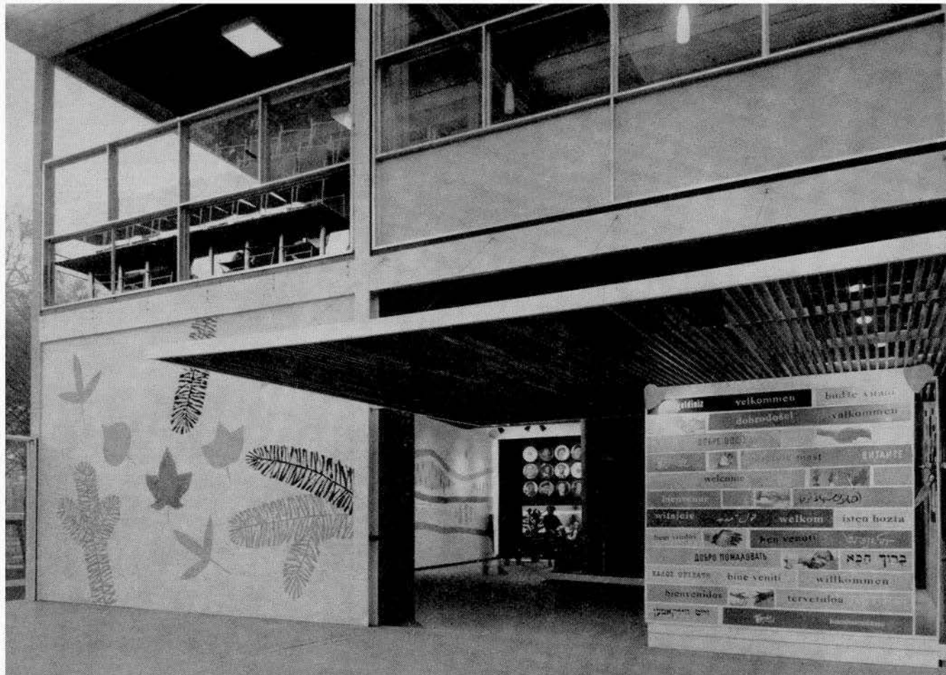
Entry to exhibition space from first floor terrace
