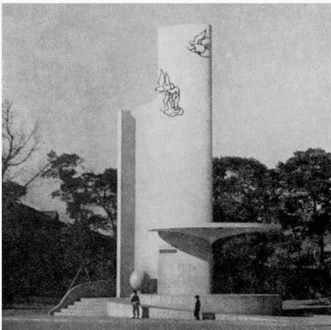
Public lavatory in playground, Tokyo
