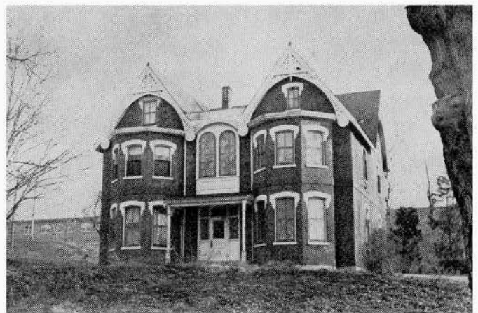
Former general hospital incorporated in the new building
