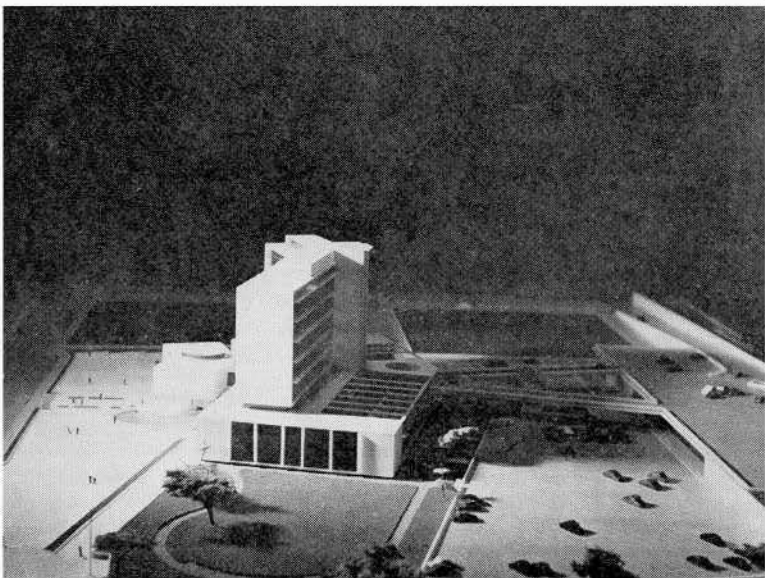
View of rear showing parking and city garage
