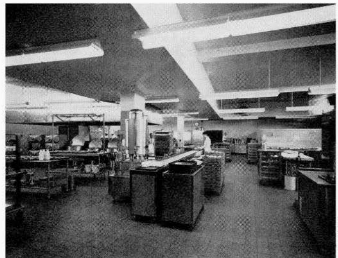
Kitchen showing reversible conveyor belt
