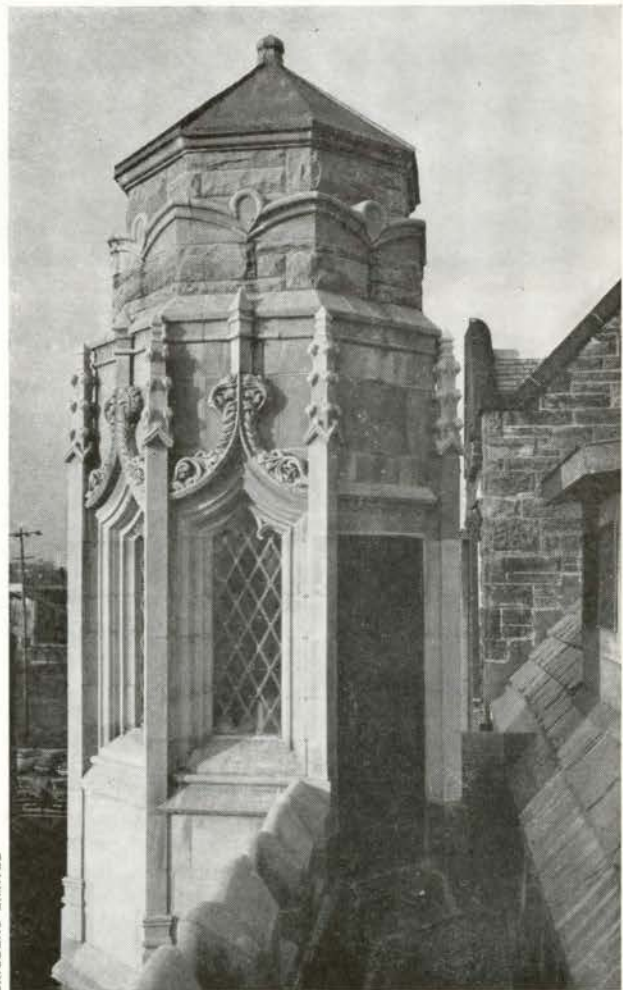
The stair turret
