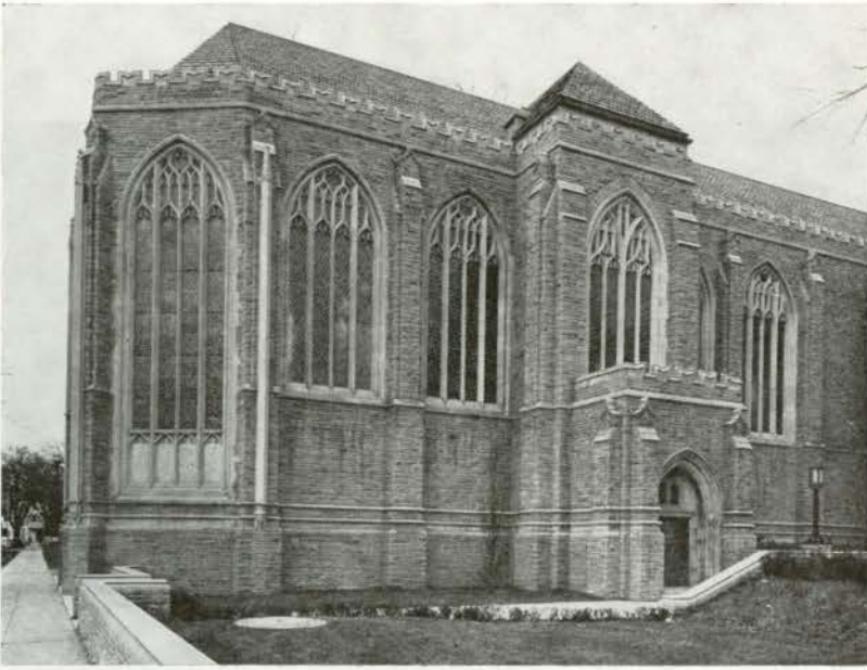
Hoskin Avenue view from the south-east
