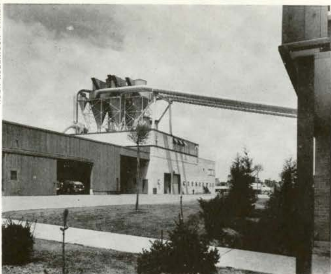
View of Boiler Plant and sawdust and shaving collection system from factory entrance
