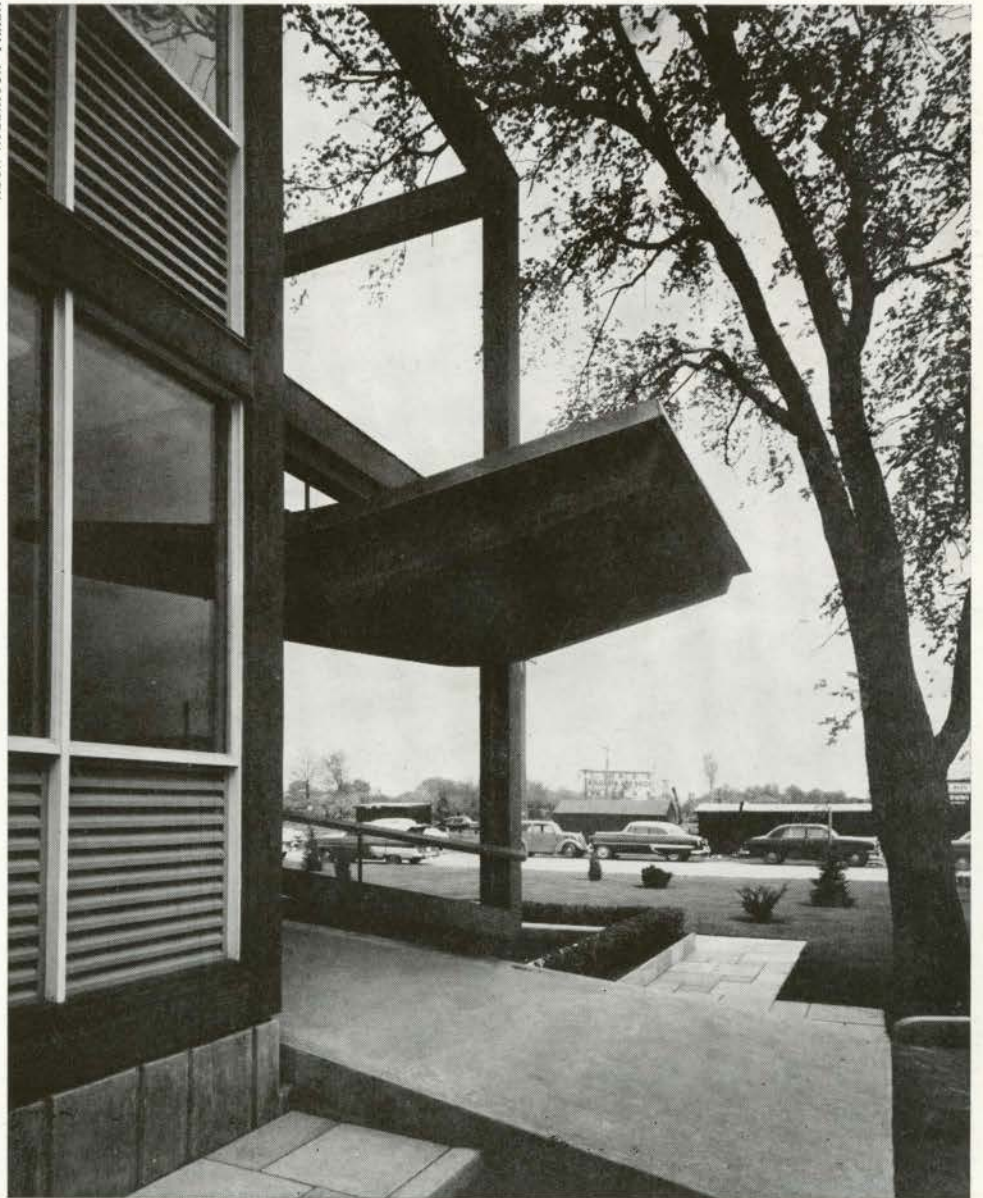
Detail of main entrance
