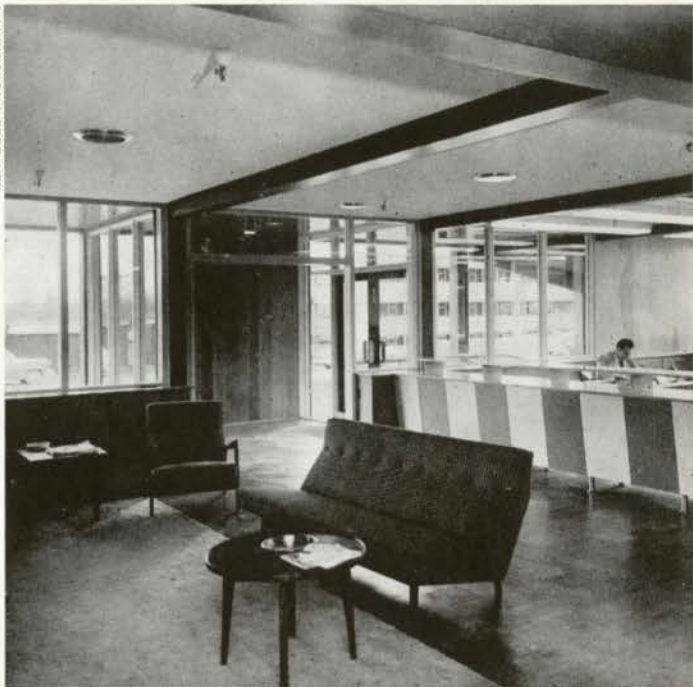
Interior of reception foyer looking towards main entrance
