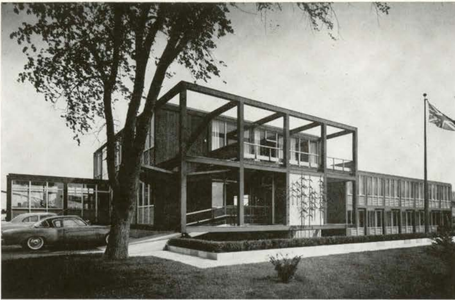
Main entrance from south
