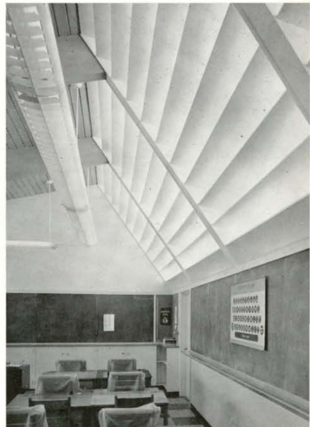
Classroom showing wood louvres
