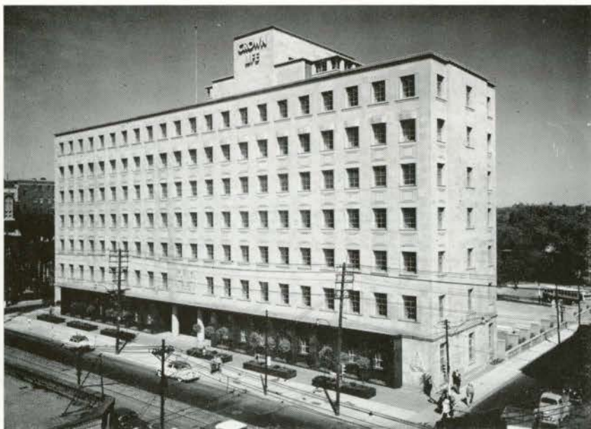
View from the south-east
