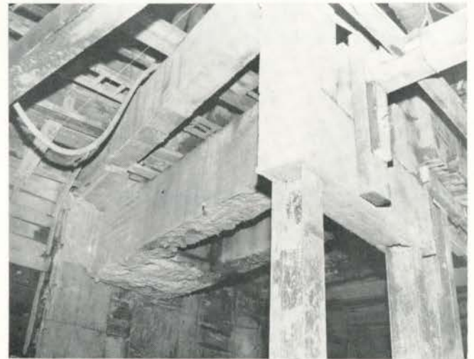
These three illustrations show underpinning of the Bank of Montreal.
