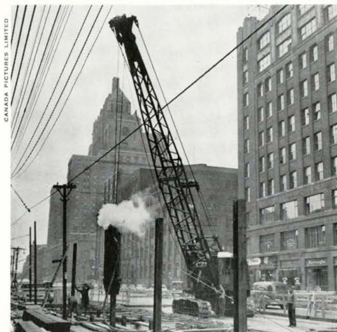
Pile driver in action
