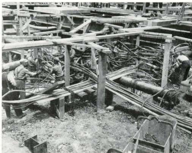
Temporary support of utilities
