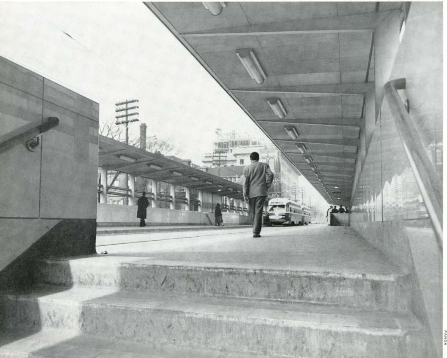
Bloor transfer platform
