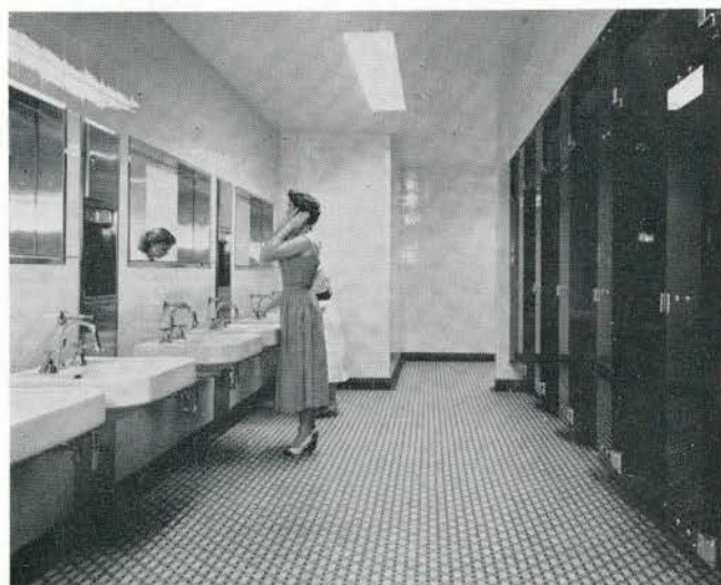
Fig. 6 View of women's typical washroom.
