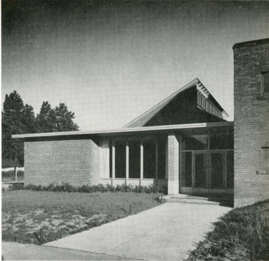
ENTRANCE FROM THE NORTH
