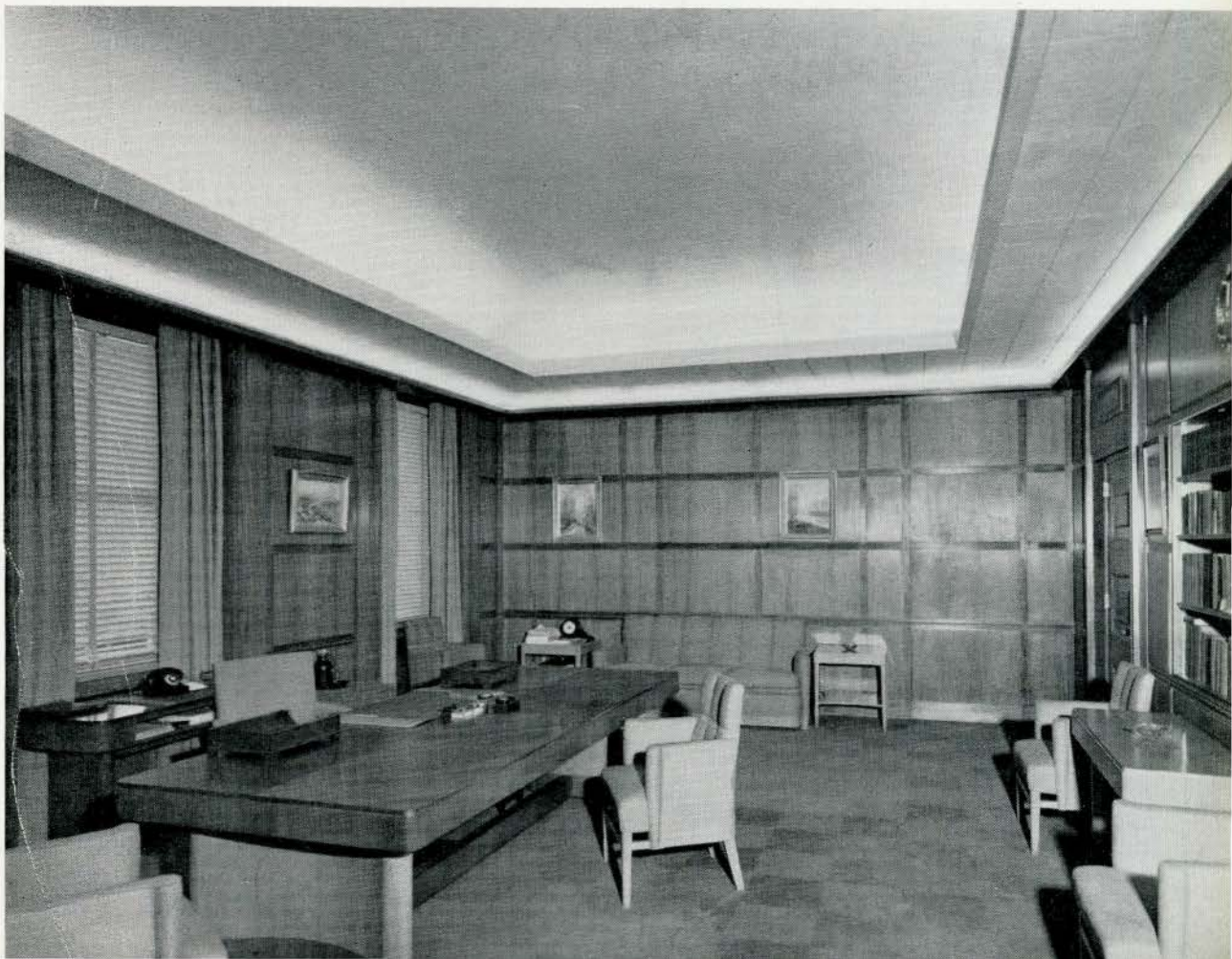
PRIVATE OFFICE ON THE THIRD FLOOR
