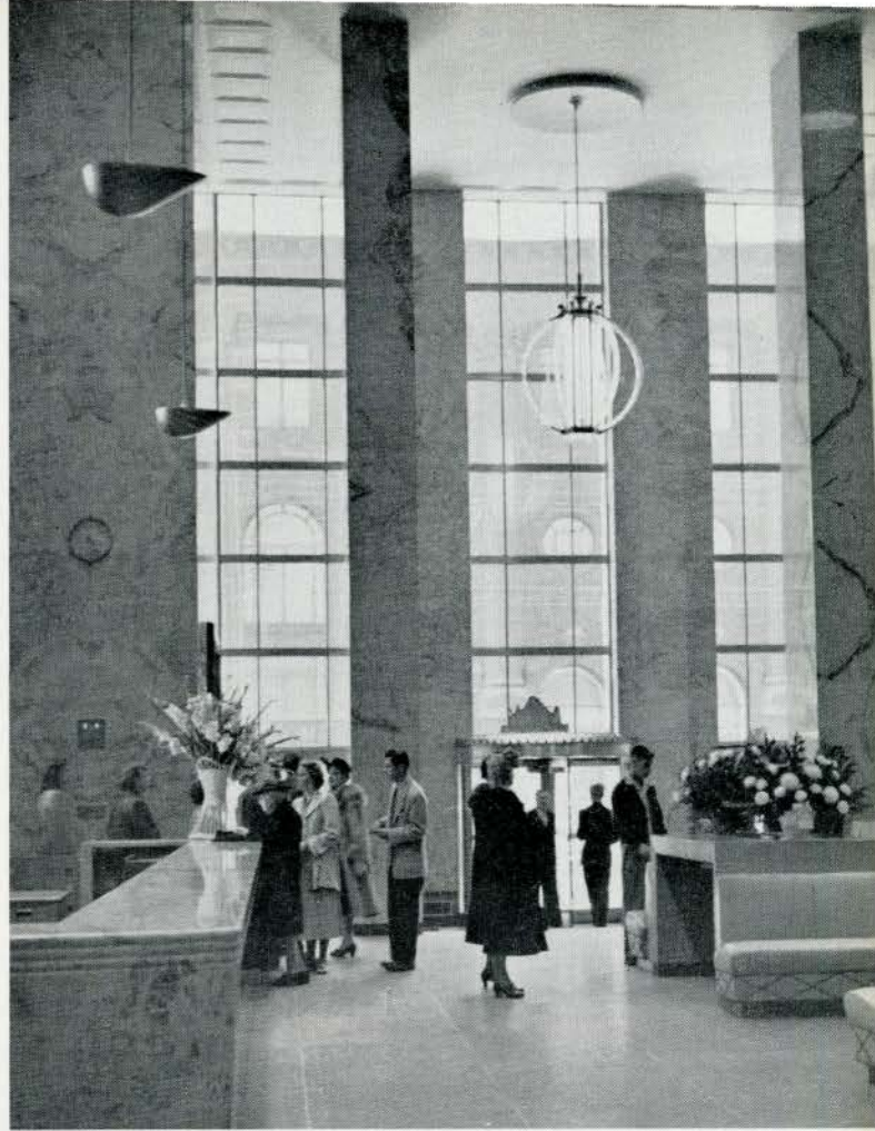
KING STREET ENTRANCE FROM MAIN BANKING ROOM
