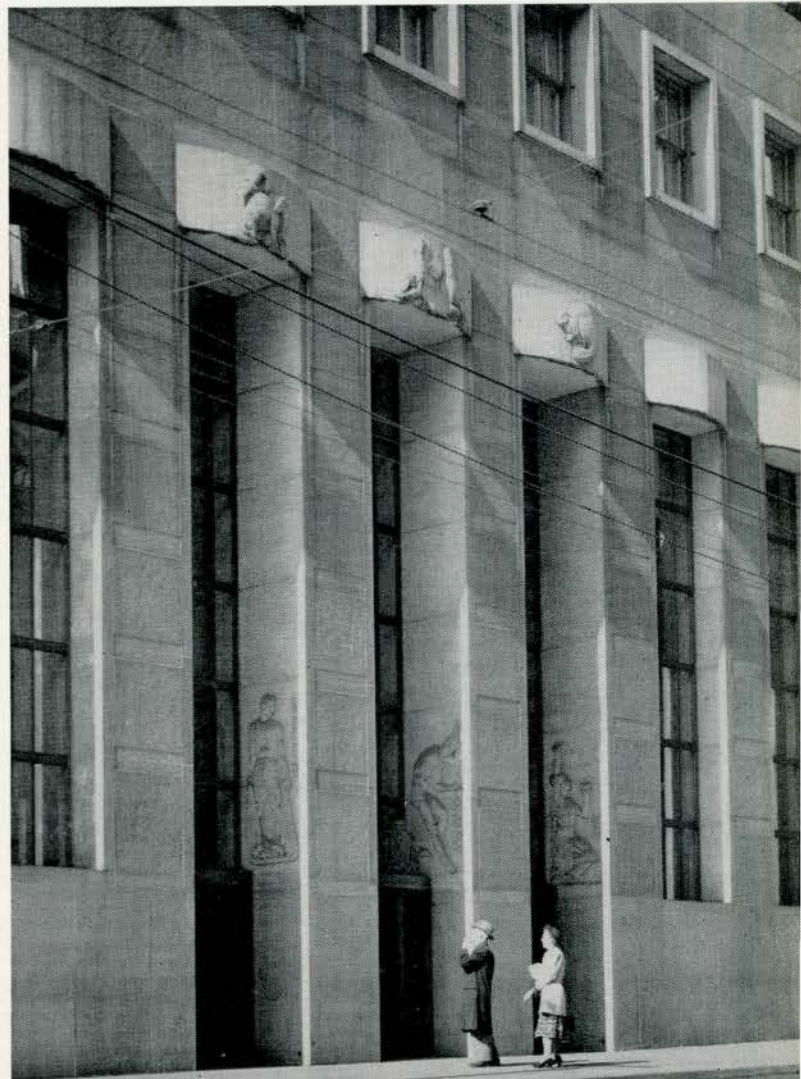
BAY STREET ENTRANCE LOOKING NORTH
