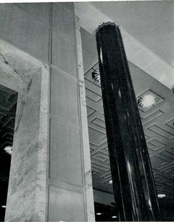
CLOSE-UP OF MARBLE COLUMN AND OAK PANELLING IN MAIN BANKING ROOM
