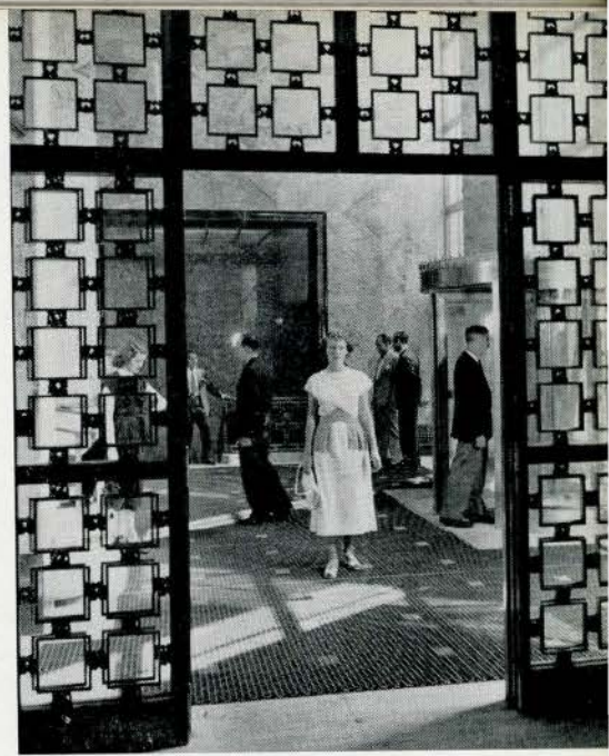
BRONZE GRILLE BETWEEN MAIN BANKING ROOM AND ELEVATOR LOBBY
