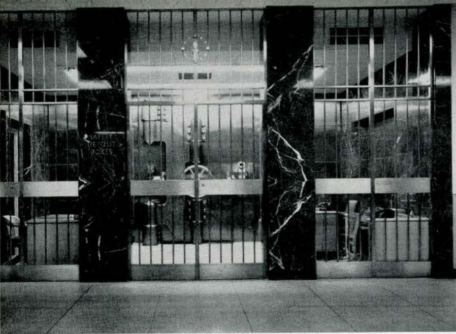
MONEL METAL GRILLE AND VAULT DOOR IN BASEMENT BANKING ROOM
