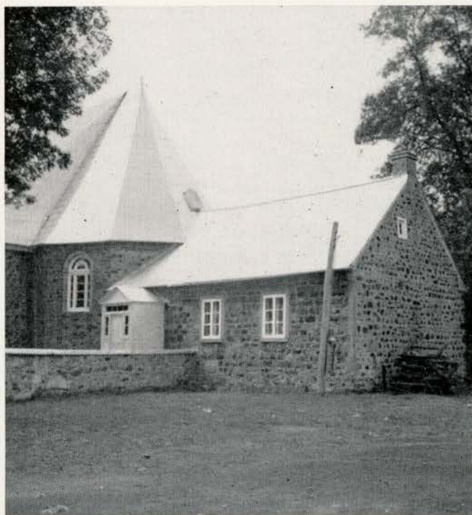
(Figure 3)—An example of apse construction en sept pans , as specified in the 1649 contract for the proposed church at Trois-Rivières. (Repentigny, ca. 1725) Phot. I.O.A.
