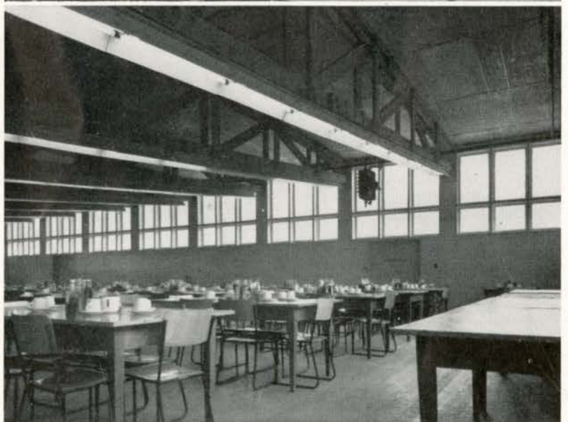
DINING ROOM SHOWING PIN POINT TRUSSES
