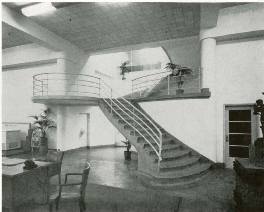
STAIR TO SECOND FLOOR OFFICES
