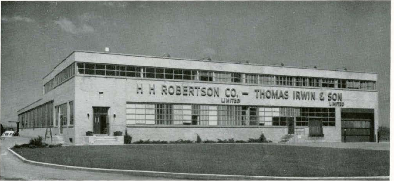
H. H. ROBERTSON CO. LIMITED — THOMAS IRWIN & SON LIMITED, HAMILTON, ONTARIO PRACK AND PRACK, ARCHITECTS
