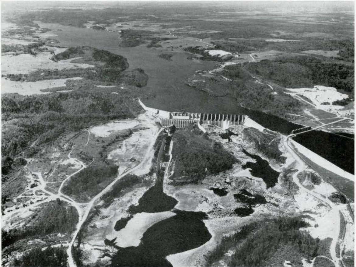
AERIAL VIEW OF SHIPSHAW NO. 1 POWERHOUSE AND DAM SHOWING CONTROL GATES AND CANAL IN CENTER RIGHT
