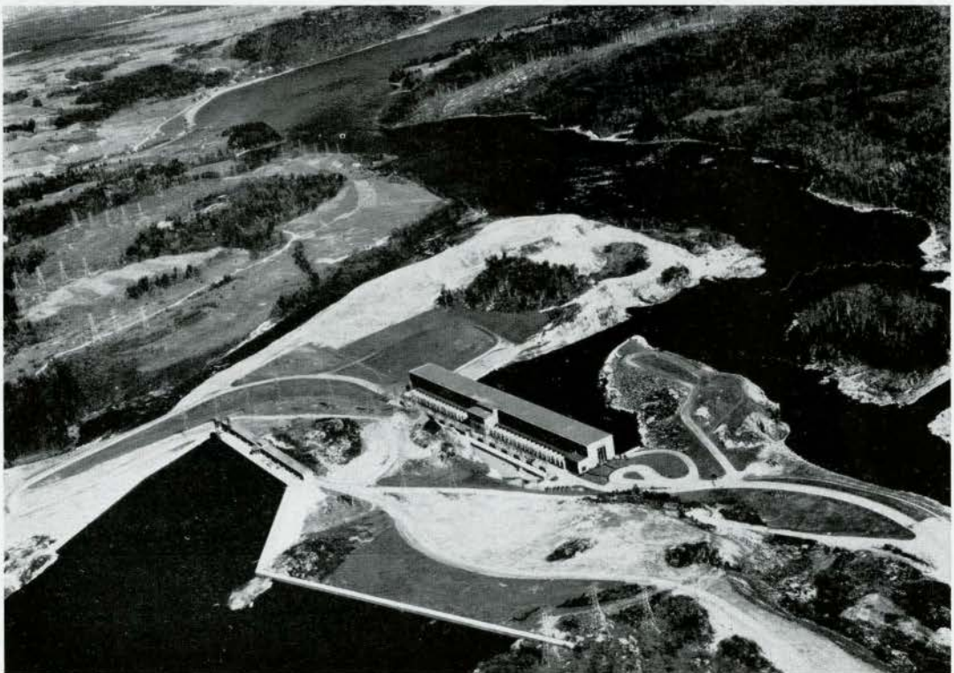
AERIAL VIEW OF SHIPSHAW NO. 2 TAKEN FROM THE REAR
