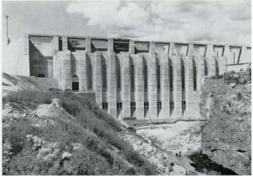
SHIPSHAW NO. 1 POWERHOUSE
