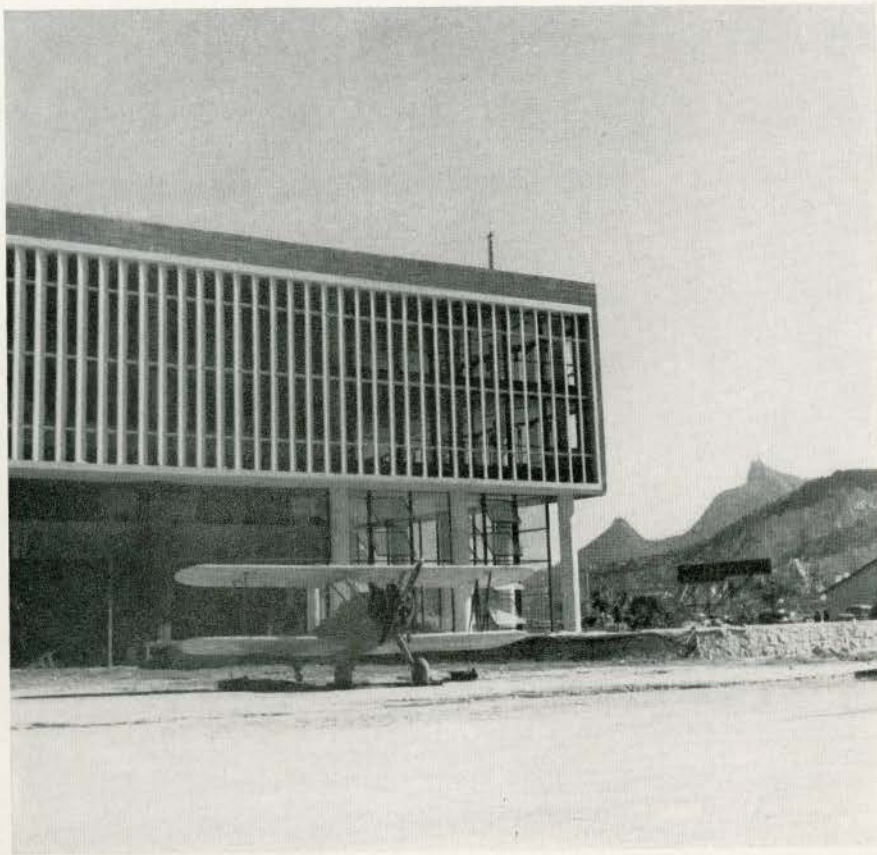
The northern façade with the completed brise-soleil.
