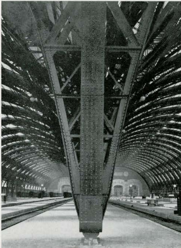
View of the platforms of the Milan terminal. An immense steel structure composed of three vaults covers the platforms. The span of the central vault is 79 yards, that of each of the side vaults 55 yards. The length of the vaults is 370 yards. This was the last station to have the complete enclosure of the platforms. Its fine engineering work fulfills at great cost a purpose which is met to-day by simple cantilevered canopies.
