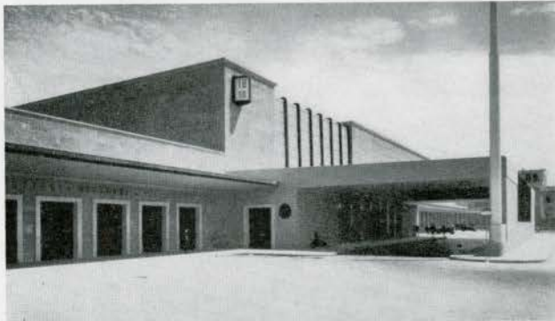
Main entrance: A band of glass slabs runs over the car canopy up the wall and over the roof to light the main lobby.
