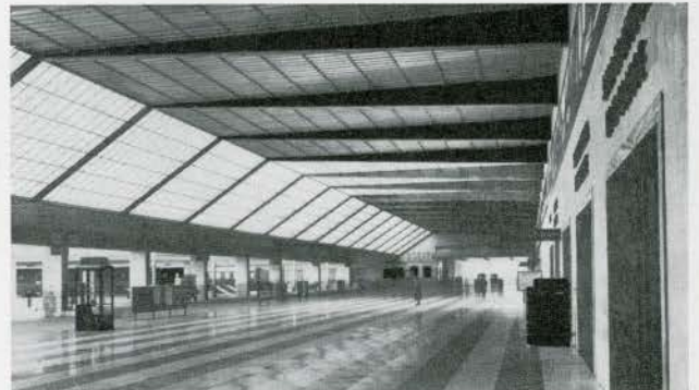
Hall leading to platforms: The band of glass slabs in the ceiling of the lobby is continued over this hall. The hall is open without doors to the platforms on the left.
