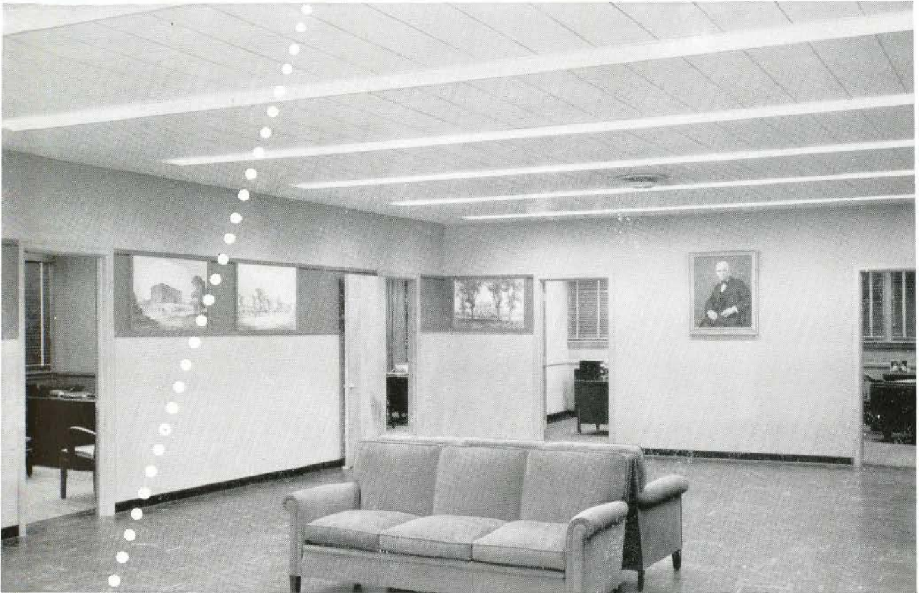
A typical example of office lighting with Curtis Fluorescent Troffers, assuring high-level, glare-free illumination for maximum eye comfort and efficiency.
