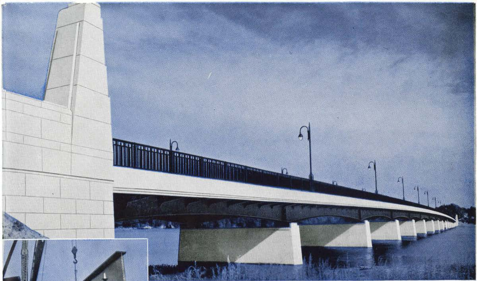
New bridge across the Rivière des Mille Îles at St. Rose, Quebec. Owners: Dept. of Public Works, Quebec. General Contractor: Dufresne Engineering Co., Ltd. Steel Fabrication and Erection: Dominion Bridge Co., Ltd. Consulting Engineers: Baulne and Leonard.
