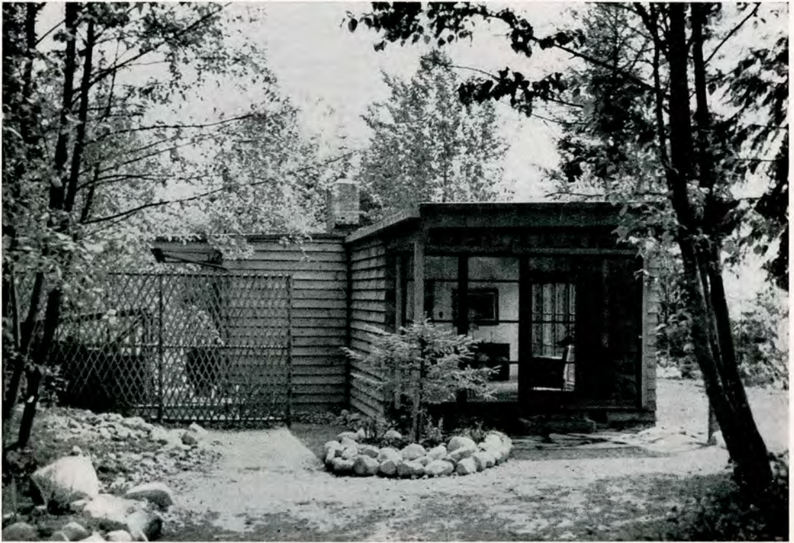
HOUSE OF MRS STUART ROSS, CAPILANO HIGHLANDS, NORTH VANCOUVER, B. C. GARDINER AND THORNTON, ARCHITECTS
