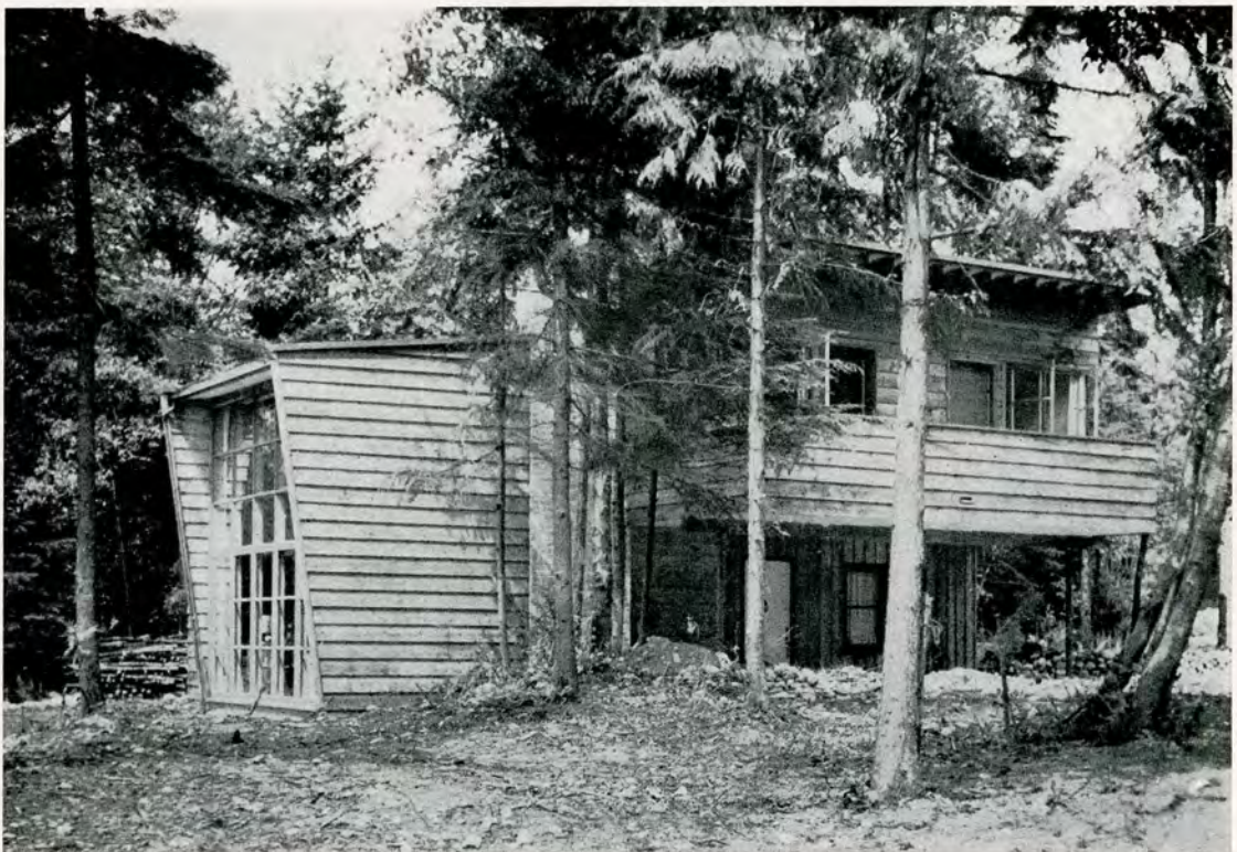
HOUSE OF MR. AND MRS. GEORGE SHERWOOD, CAPILANO HIGHLANDS, NORTH VANCOUVER, B. C. GARDINER AND THORNTON, ARCHITECTS
