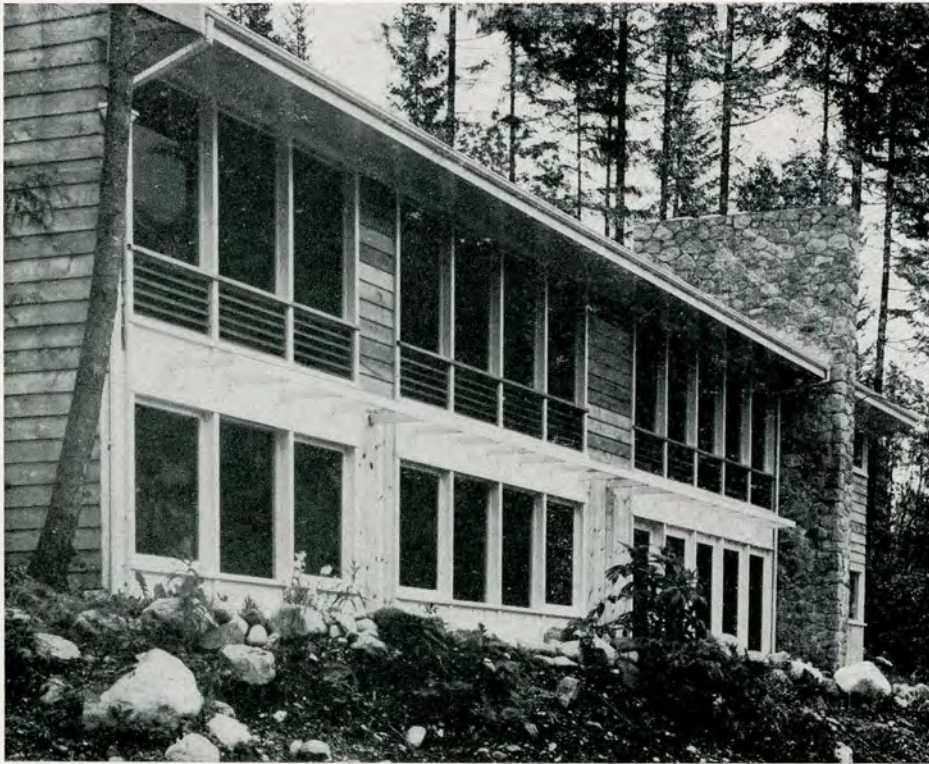
SPECULATIVE HOUSE AT GLEN EAGLES PARK, WEST VANCOUVER, B. C. SHARP & THOMPSON, BERWICK, PRATT, ARCHITECTS
