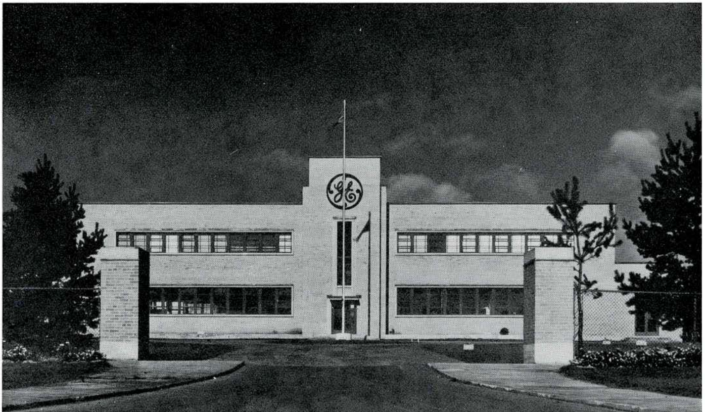
CANADIAN GENERAL ELECTRIC COMPANY LIMITED, SMALL APPLIANCE PLANT, BARRIE, ONTARIO
