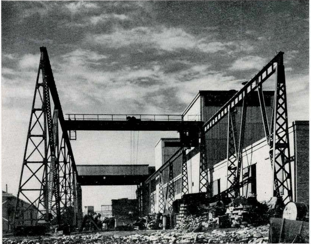
SOUTH SIDE LOOKING WEST
