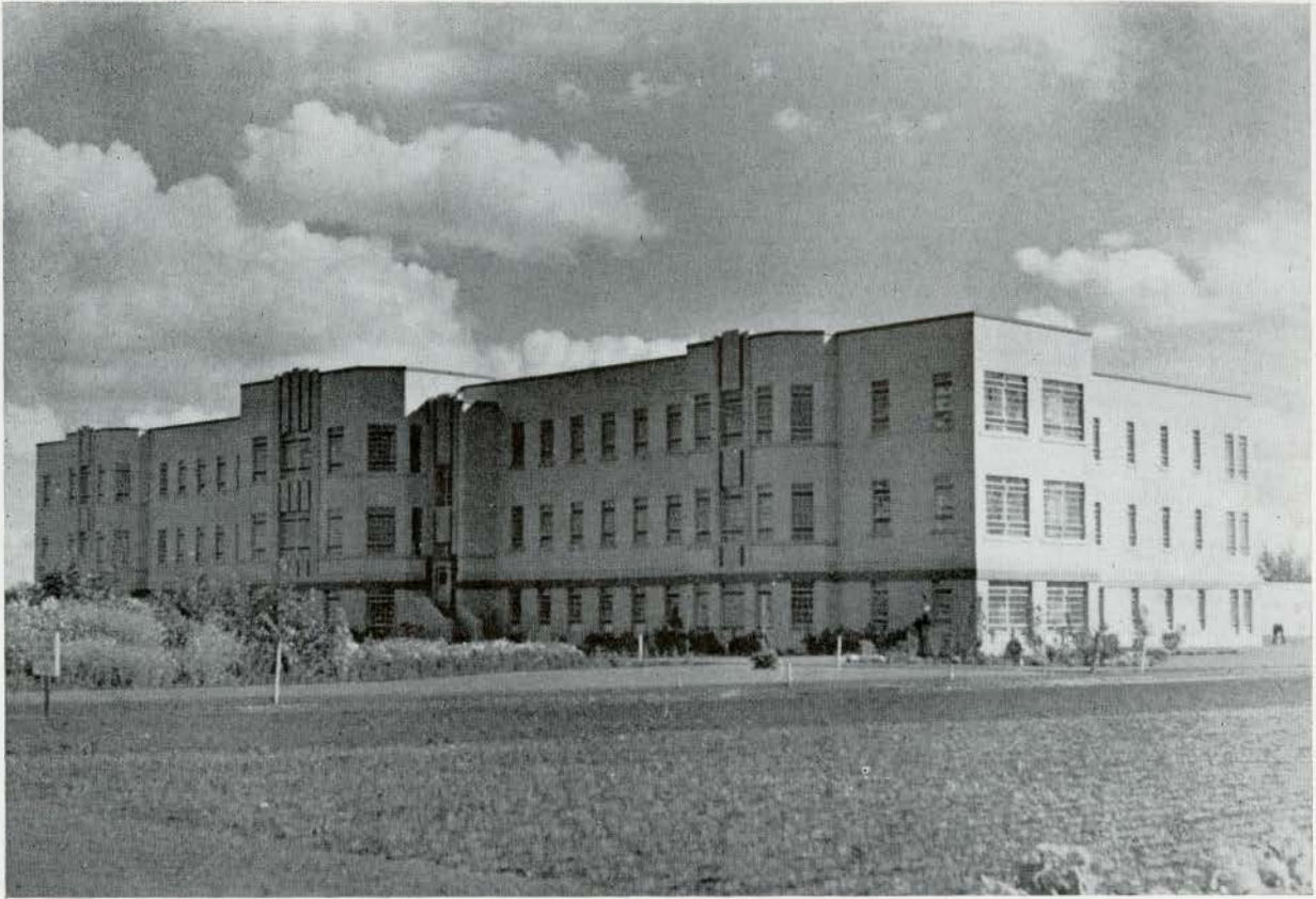
DORMITORY NO. 5, PROVINCIAL MENTAL INSTITUTE, OLIVER, ALBERTA BUILDING BRANCH, DEPARTMENT OF PUBLIC WORKS
