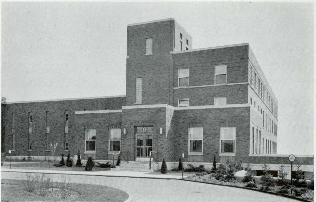
QUEEN ELIZABETH PAVILION, BRANTFORD GENERAL HOSPITAL, BRANTFORD, ONTARIO
