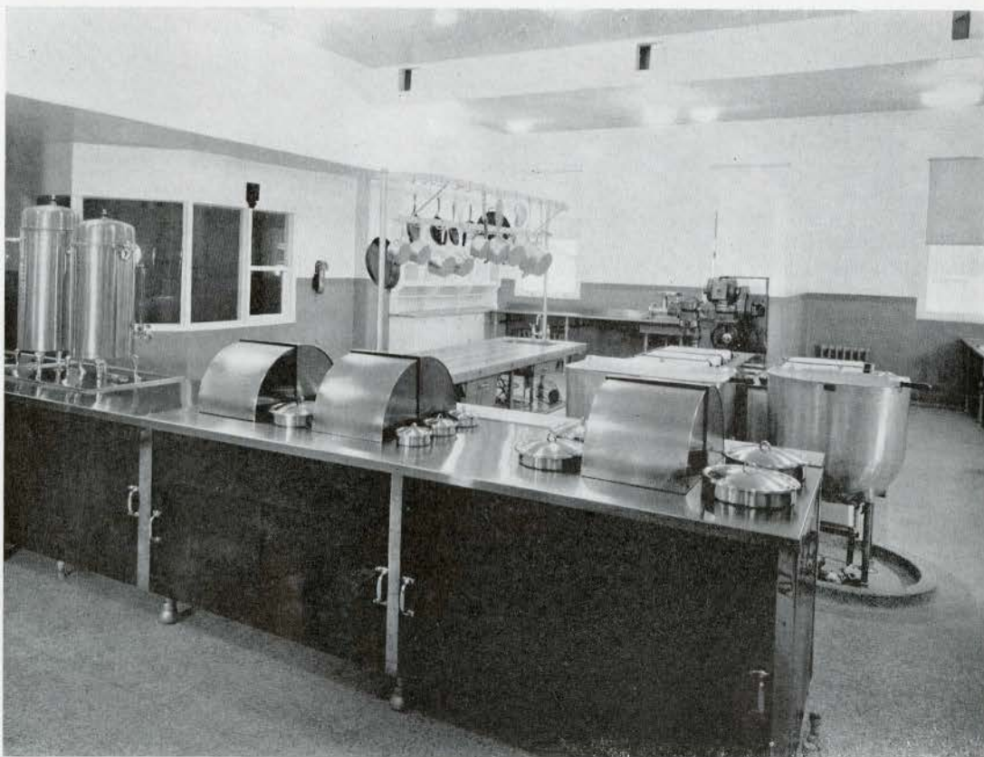
PART OF MAIN KITCHEN, OSHAWA GENERAL HOSPITAL, OSHAWA, ONTARIO
