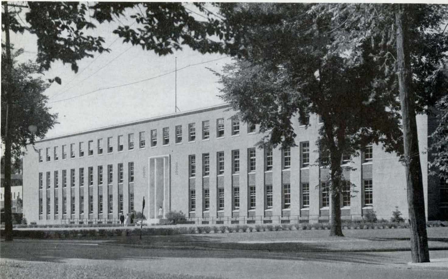
KING EDWARD AVENUE BUILDING, BANK OF CANADA, OTTAWA, ONTARIO MARANI AND MORRIS, ARCHITECTS
