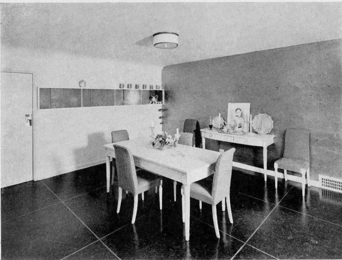
Dining room showing built in china cupboard.
