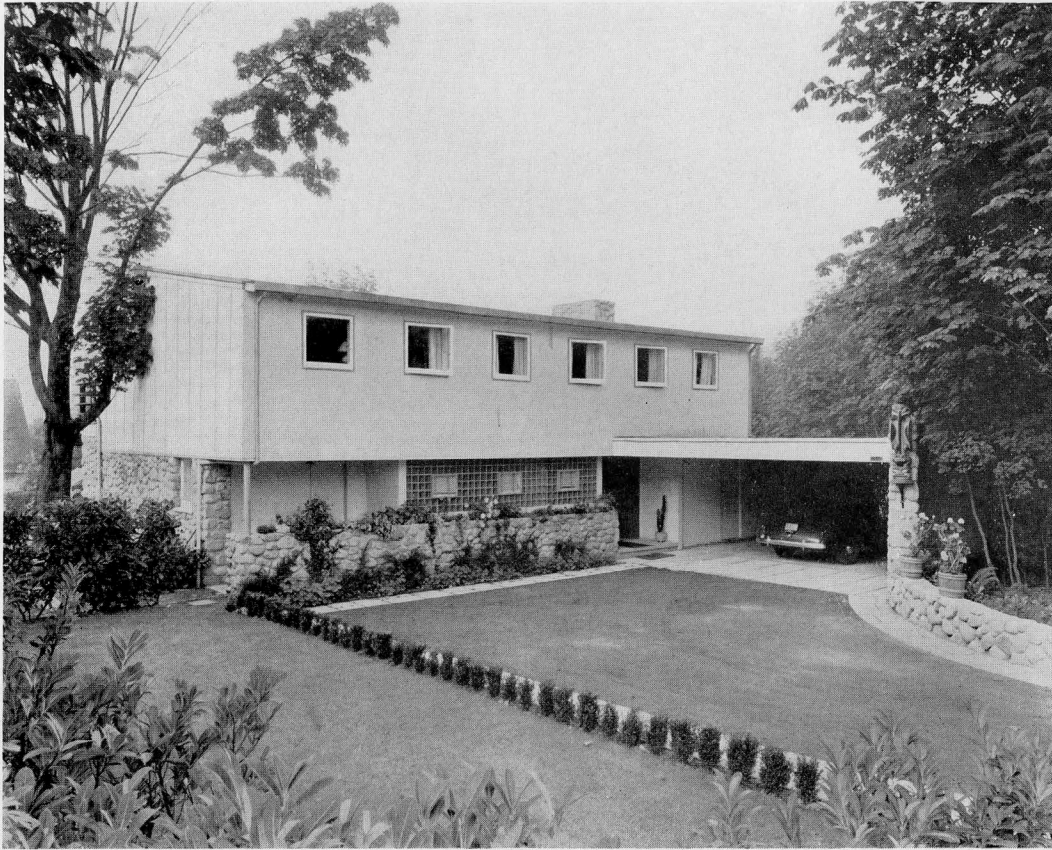
North elevation showing driveway and open garage with totem pole motif, typical of British Columbia native craftsmanship. The house is built of boulder stone and white plywood vertical siding. The trim around the windows is painted peach.
