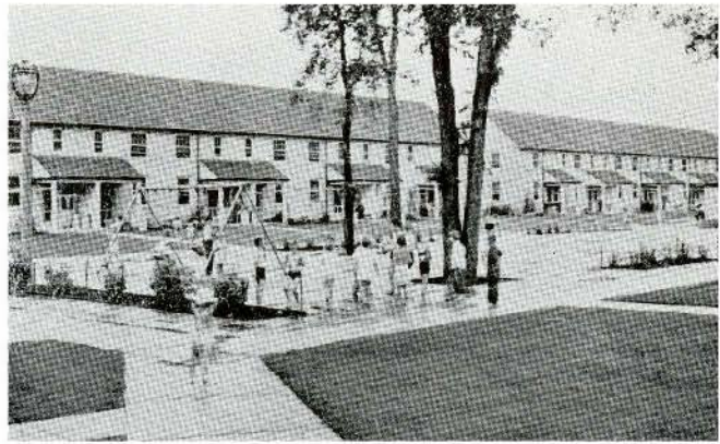
12. GOOD HOUSING, such as that at Parklawn, Milwaukee, faces inwards upon the Green and its communal institutions. Irrelevant traffic is circulated around the outside of its domestic privacy. It was built by the Federal government and is operated by the local Housing Authority. Such projects are bulwarks against the alarming decline in the urban birth-rate.
