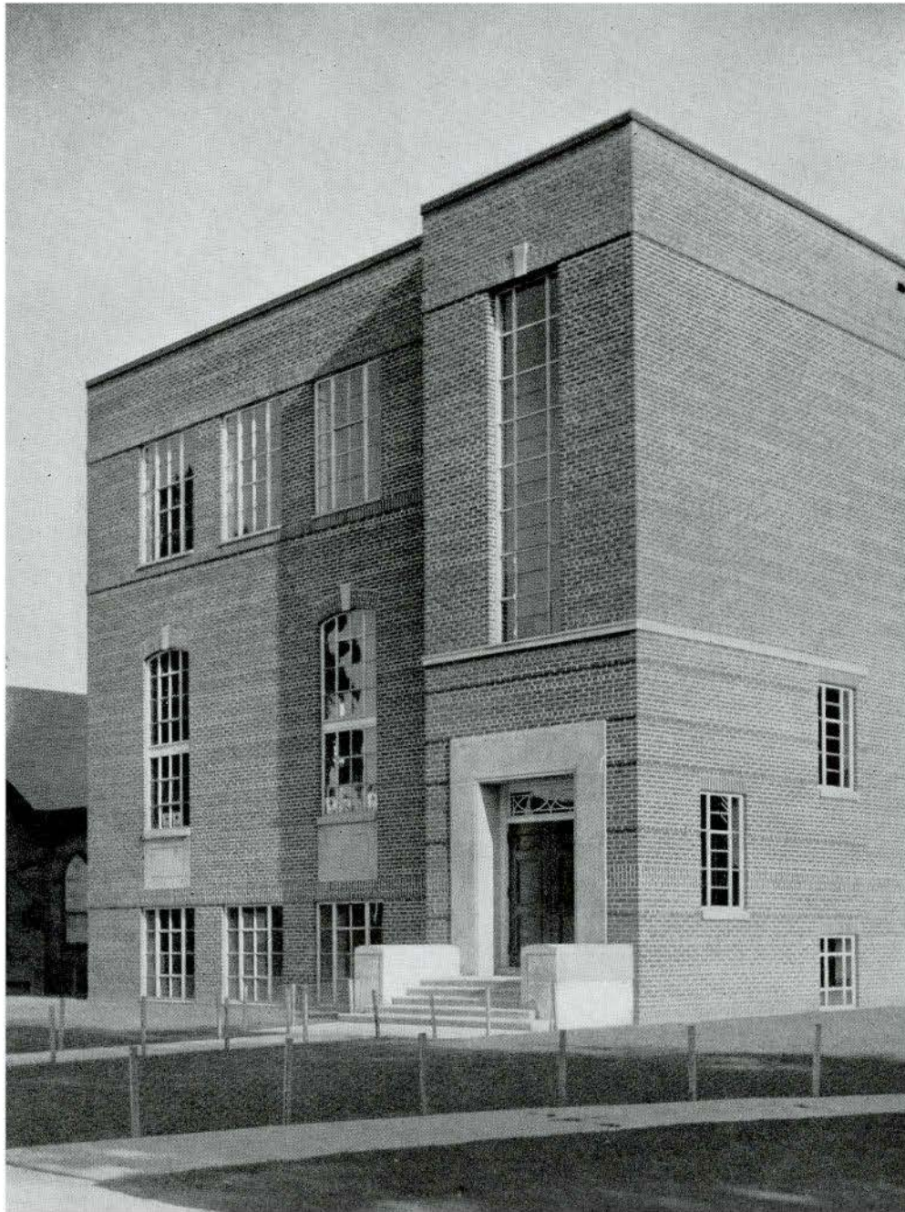
ADDITION TO THE COLLEGIATE INSTITUTE, COBOURG, ONTARIO S. B. COON AND SON, ARCHITECTS
