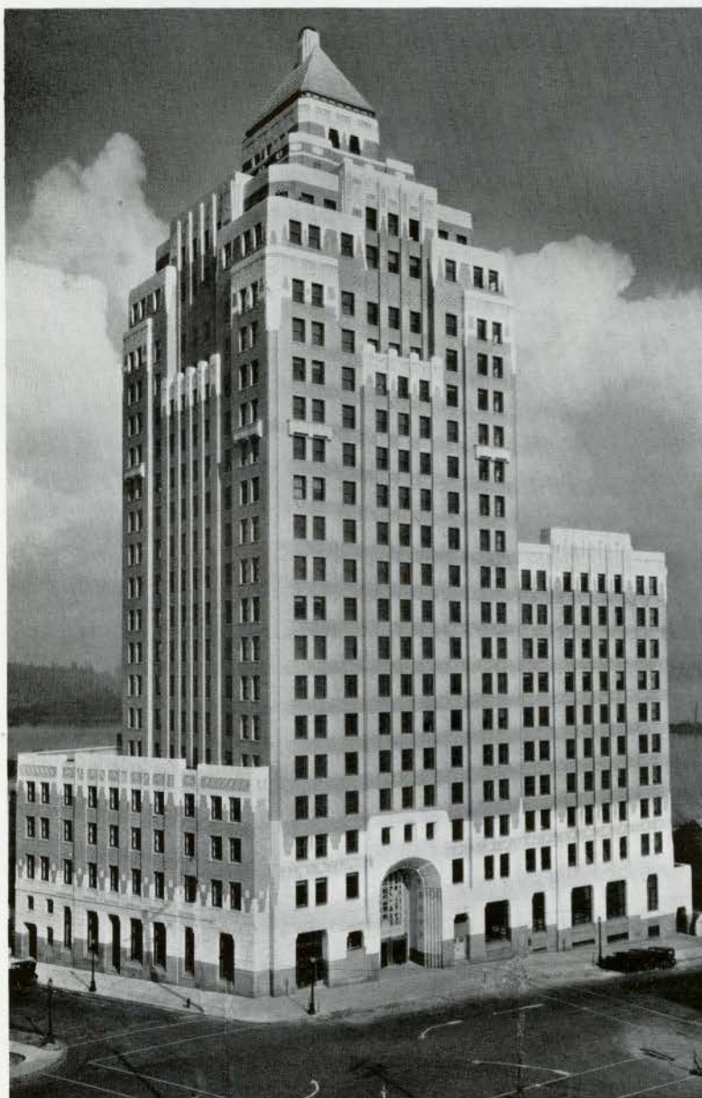
Marine Bldg., Vancouver, B.C. McCarter & Nairne, architects; Leek & Company, Ltd., mechanical contractors, Vancouver. Heating and ventilating systems for stock exchange and banking areas are Johnson-controlled.
