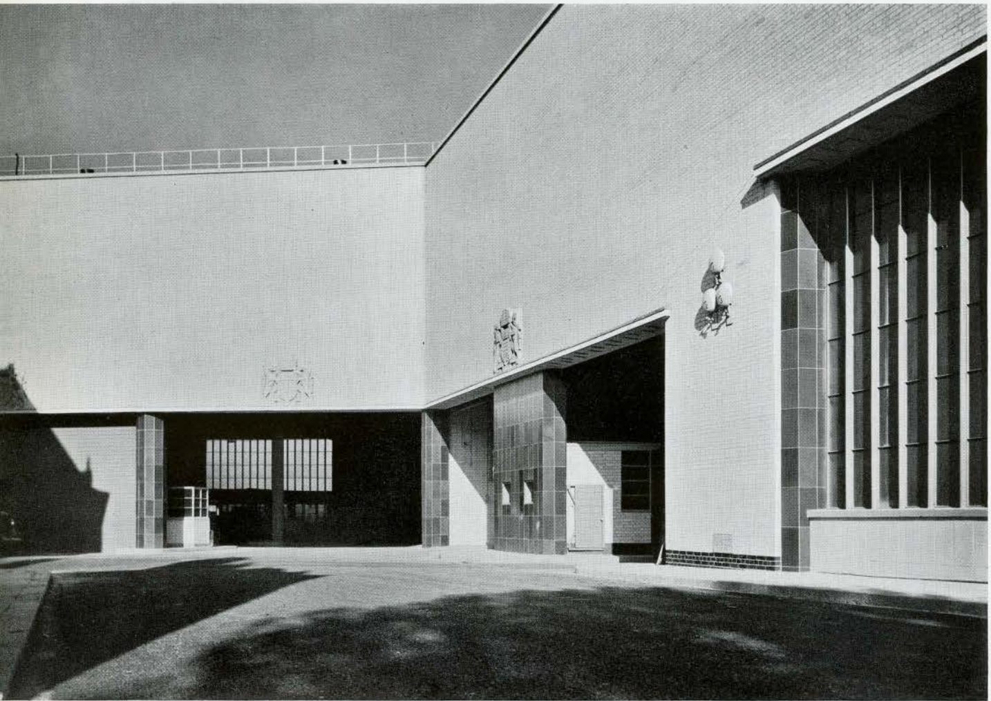
CENTRAL CLEANSING AND TRANSPORT DEPOT FOR THE CITY OF WESTMINSTER, ENGLAND LONDON ARCHITECTURE MEDAL AWARD GREY WORNUM, ARCHITECT LIONEL SMITH, ASSISTANT
