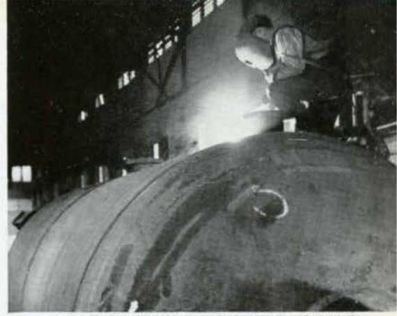
• ELECTRIC ARC WELDING •
