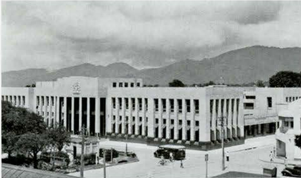
TREASURY AND POST OFFICE BUILDING, PORT OF SPAIN
