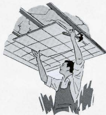
Overhead work is simplicity itself with this easy-to-handle sheet material. Can be nailed right over cracked plaster on furring strips.
