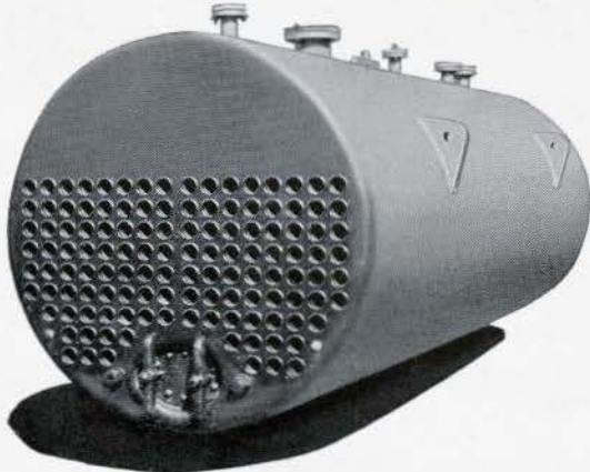
Welded H.R.T. Boiler in Queen's Hotel, Montreal
