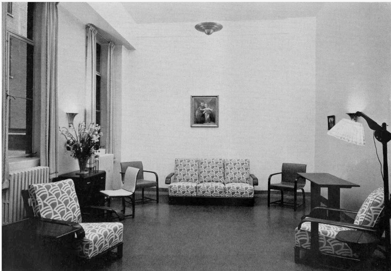
VISITORS' WAITING ROOM
