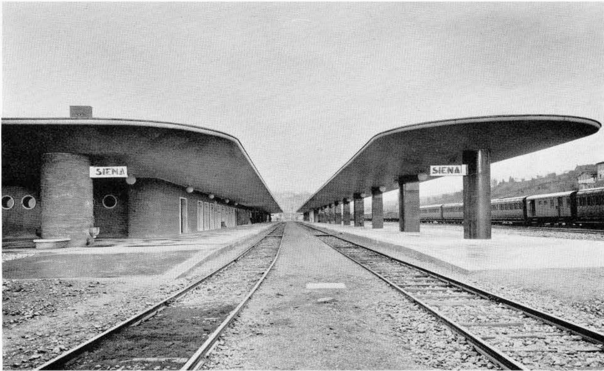
VIEW OF PLATFORM Rose Coloured Glass Canopy and Stone Columns
