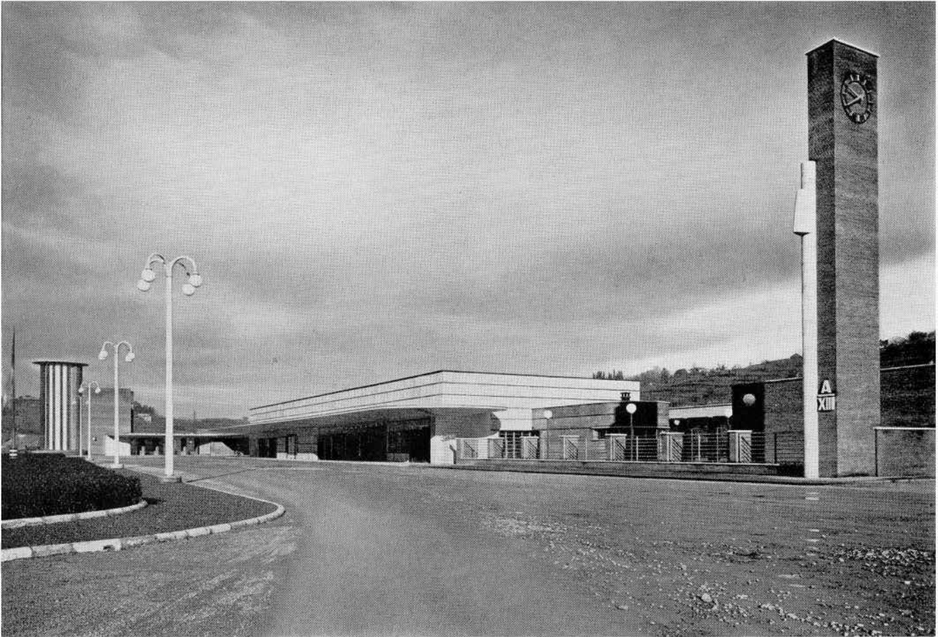
COMBINED RAILWAY STATION FOR SIENA AND REGGIO EMILIA ANGIOLO MAZZONI, ARCHITECT
