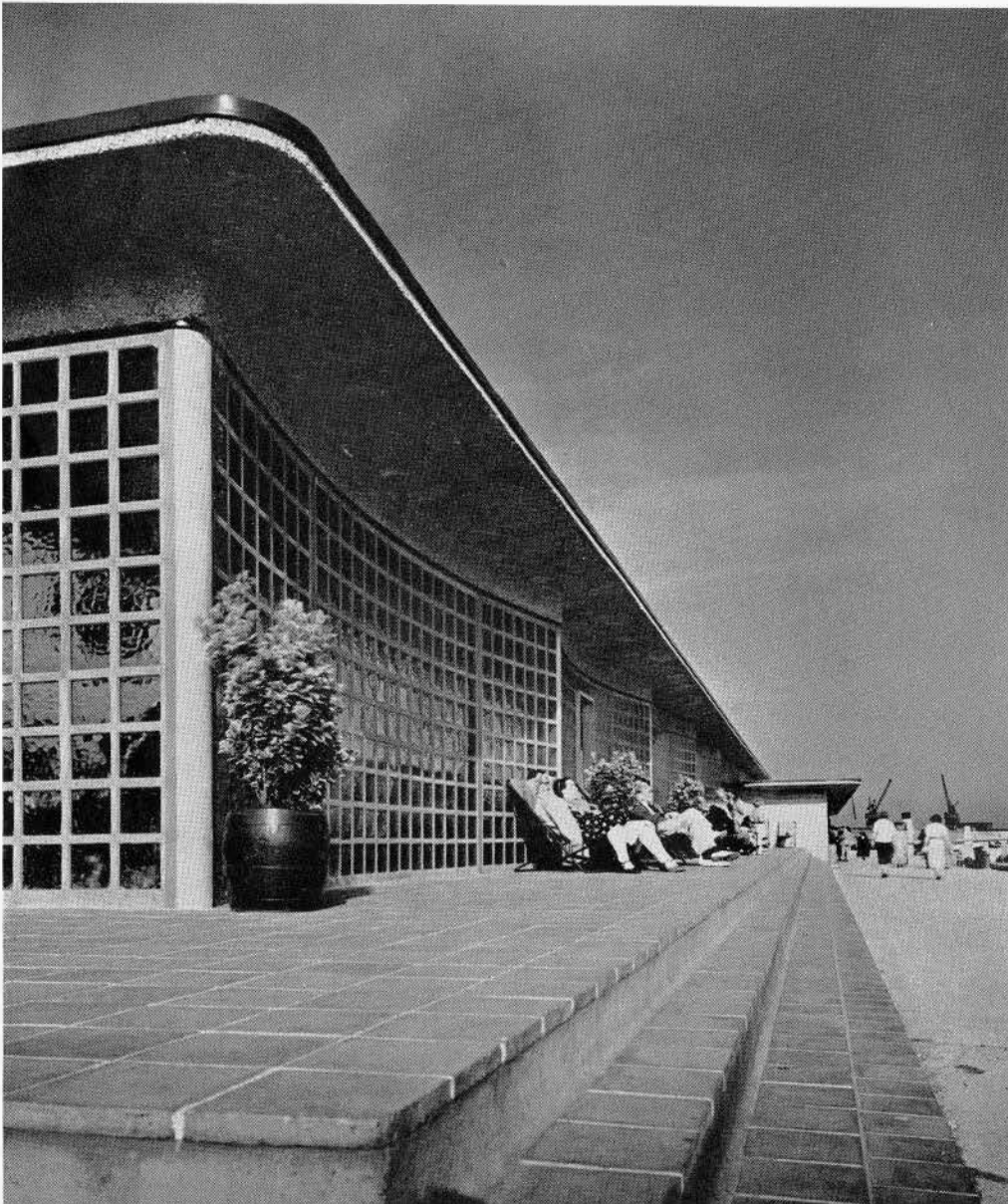
The shelter, looking along the seaward side. It is composed of a series of curved bays of concrete and glass, with a reinforced concrete roof, and is mounted on a quarry-tile platform and steps.
