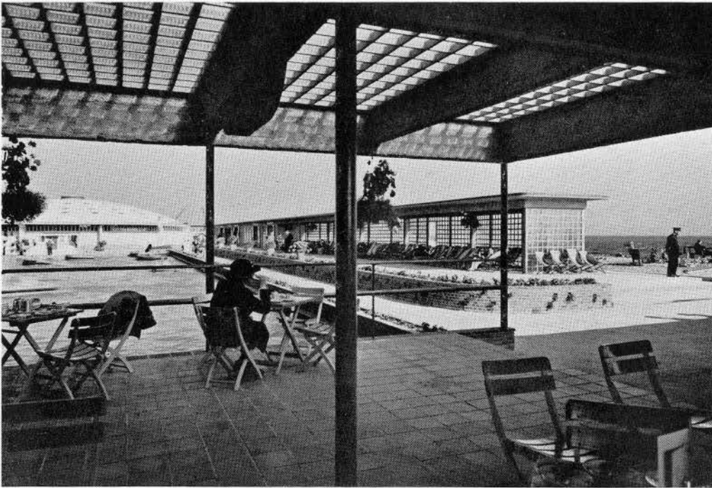
A view from the wide verandah of the restaurant at the west end of the pool, showing the whole length of the shelter and shops on the right (or south side) and the axially placed "fun-fair" rotunda at the east end.
