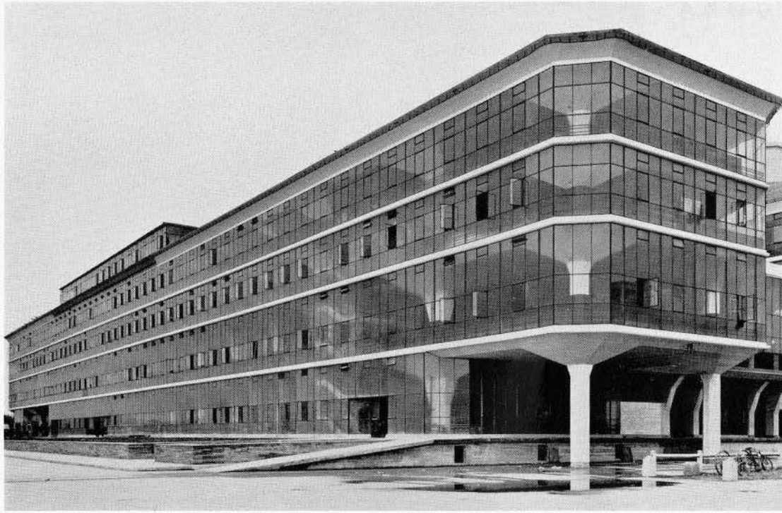
Factory for "Boots", Nottingham, designed by Sir Owen Williams. An early example of English reinforced concrete showing the lightness of appearance possible.
