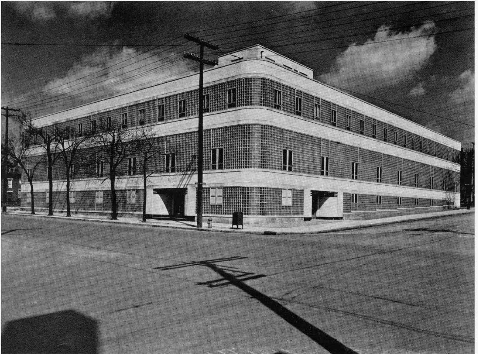
THE NEW AMERICAN EDUCATION PRESS BUILDING, COLUMBUS, OHIO
