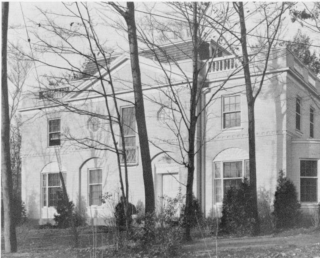
RESIDENCE OF N. R. FIRSTBROOK, ESQ., TORONTO Bruce H. Wright, M.R.A.I.C., Architect
