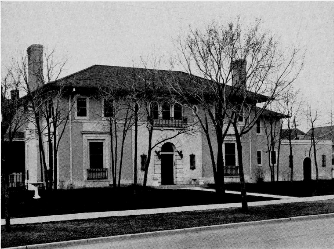
RESIDENCE OF N. J. BREEN, ESQ., WINNIPEG A. E. Cubbage, M.R.A.I.C., Architect
