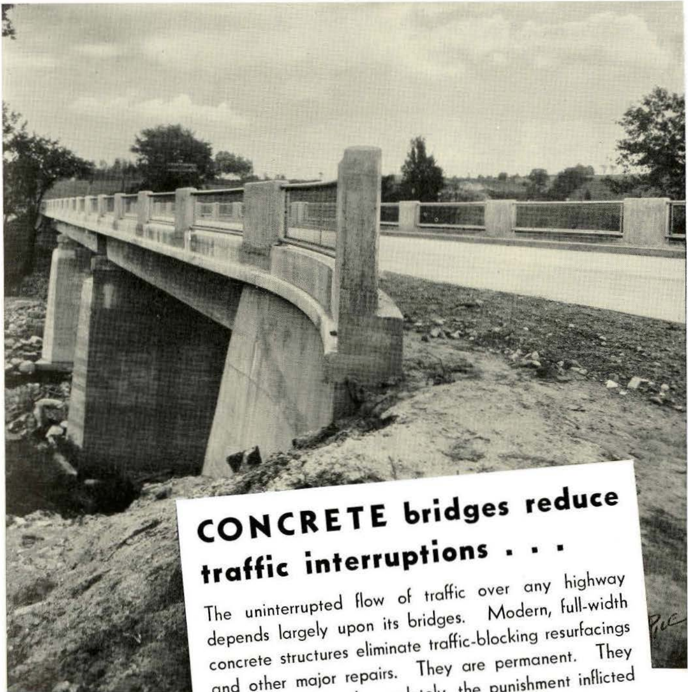
Bridge over Coaticook River on Waterville-Derby Line Highway near Sherbrooke, Que. Dept. of Public Works & Mines, Province of Quebec, J. N. Francoeur, Minister. O. Desjardins, Chief Engineer. J. P. Lachapelle, Contractor.
