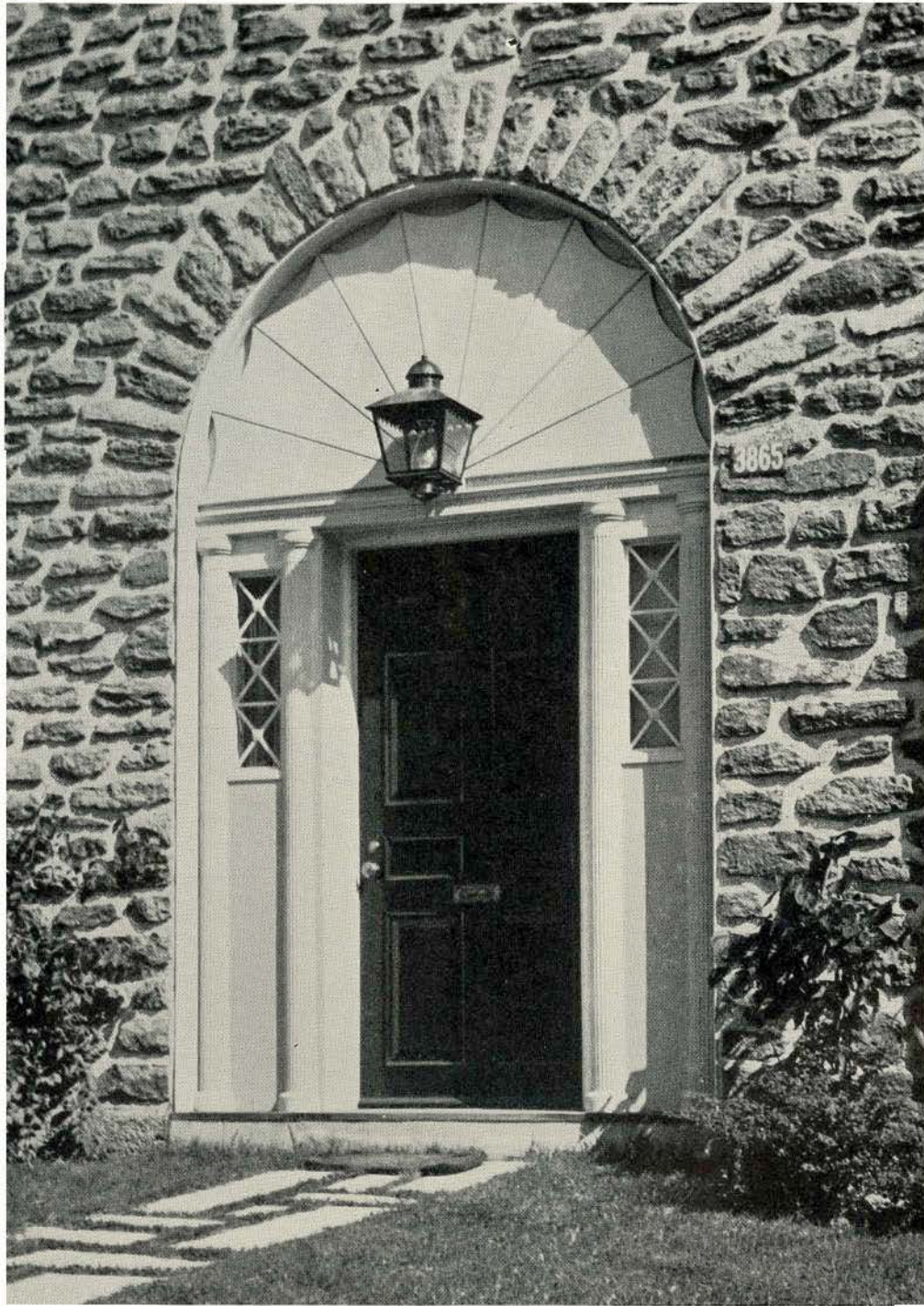
ENTRANCE DETAIL—RESIDENCE OF TREVOR ROSS, ESQ., MONTREAL
