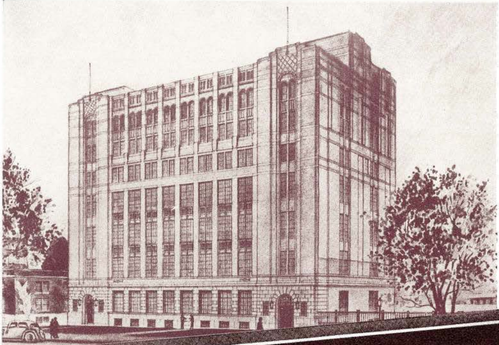
At Right—New Postal Terminal Building, Ottawa (Cecil Burgess, architect). Steelwork fabricated by Dominion Bridge Co. Ltd., using Algoma beams and channels up to 15-in. depth. The first building erected in Canada using structural sections of this size made in Canada.
