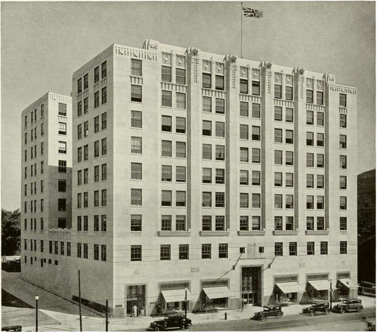
VIEW OF THE TORONTO HYDRO-ELECTRIC BUILDING FROM THE SOUTH-WEST
