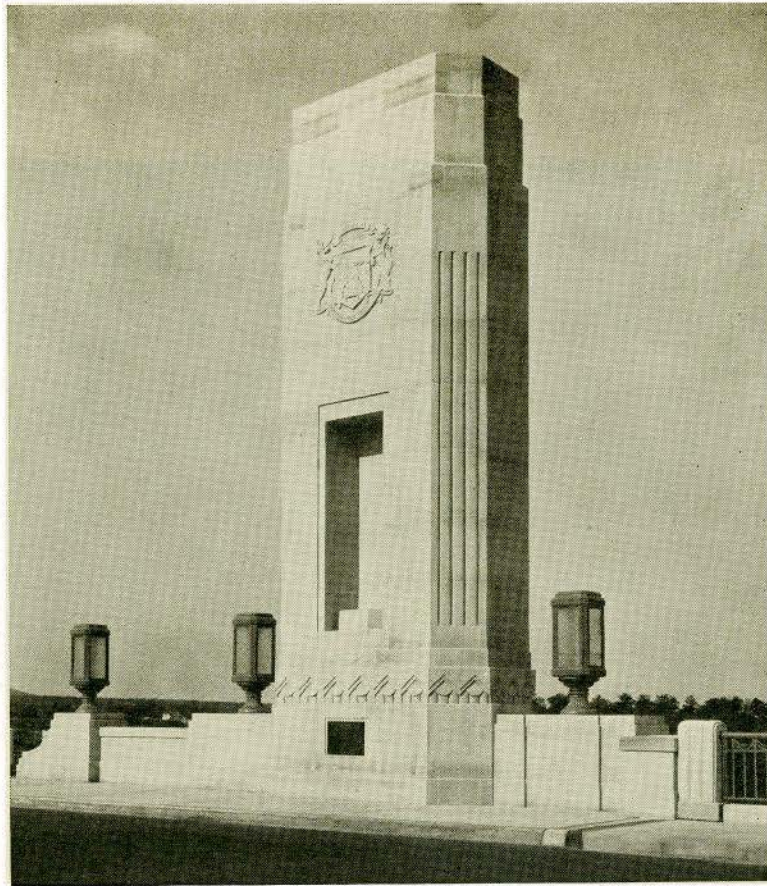
PYLON—HIGH LEVEL BRIDGE, HAMILTON
