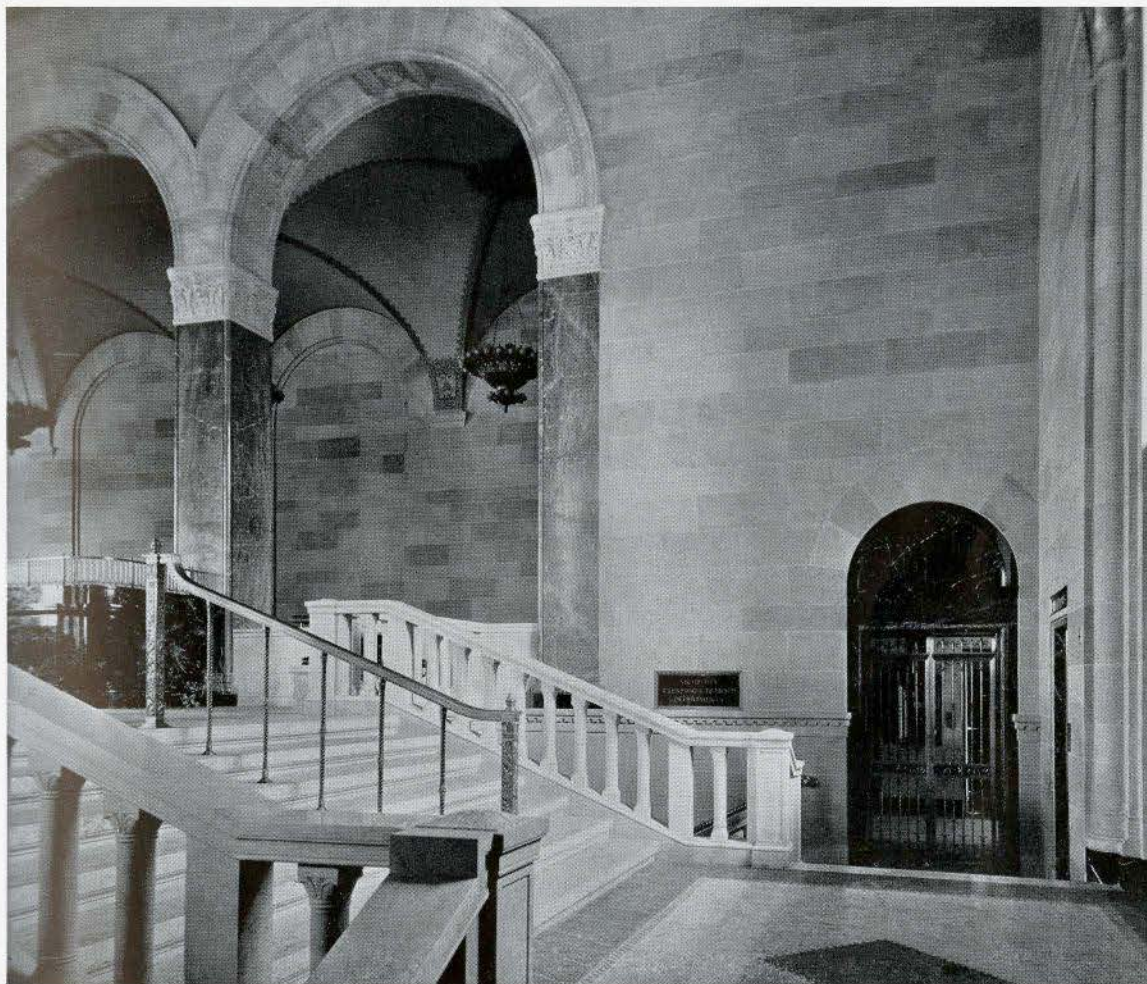
STAIRWAY TO MAIN BANKING ROOM
