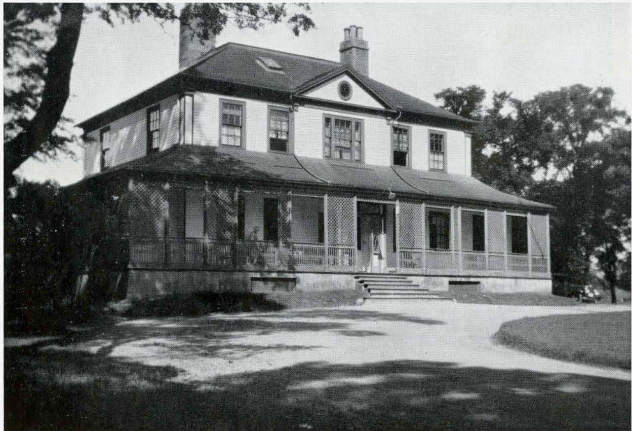
VIEW FROM THE DRIVEWAY
