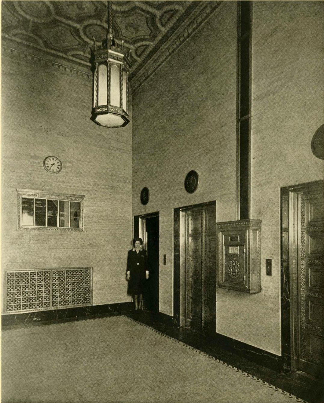
ELEVATOR HALL—ROYAL BANK BUILDING, VANCOUVER S. G. Davenport, Architect
