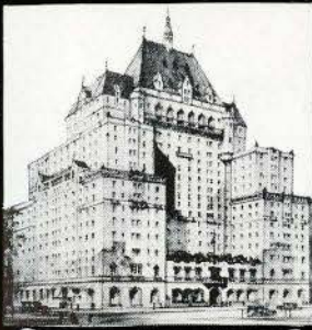
Canadian National Hotel Vancouver John S. Archibald and John Schofield Associate Architects
