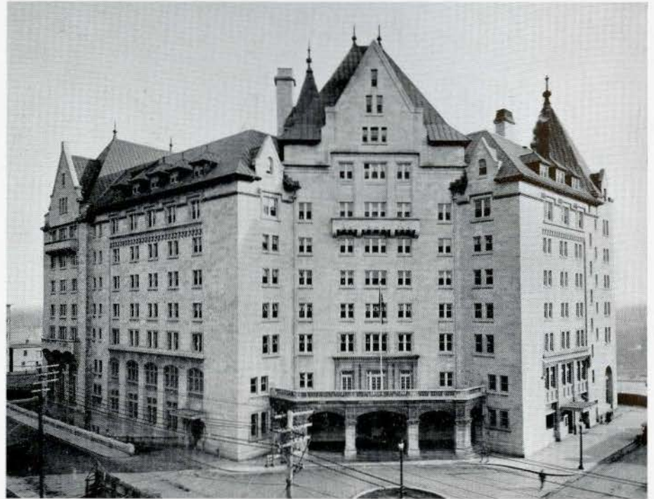
• The Macdonald Hotel Edmonton, Alta. Architects—Ross & Macdonald •
