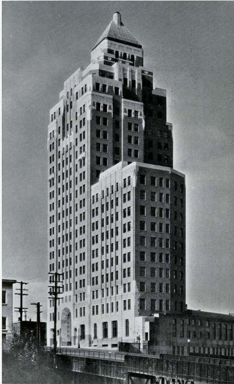
VIEW OF THE MARINE BUILDING FROM THE WATERFRONT
