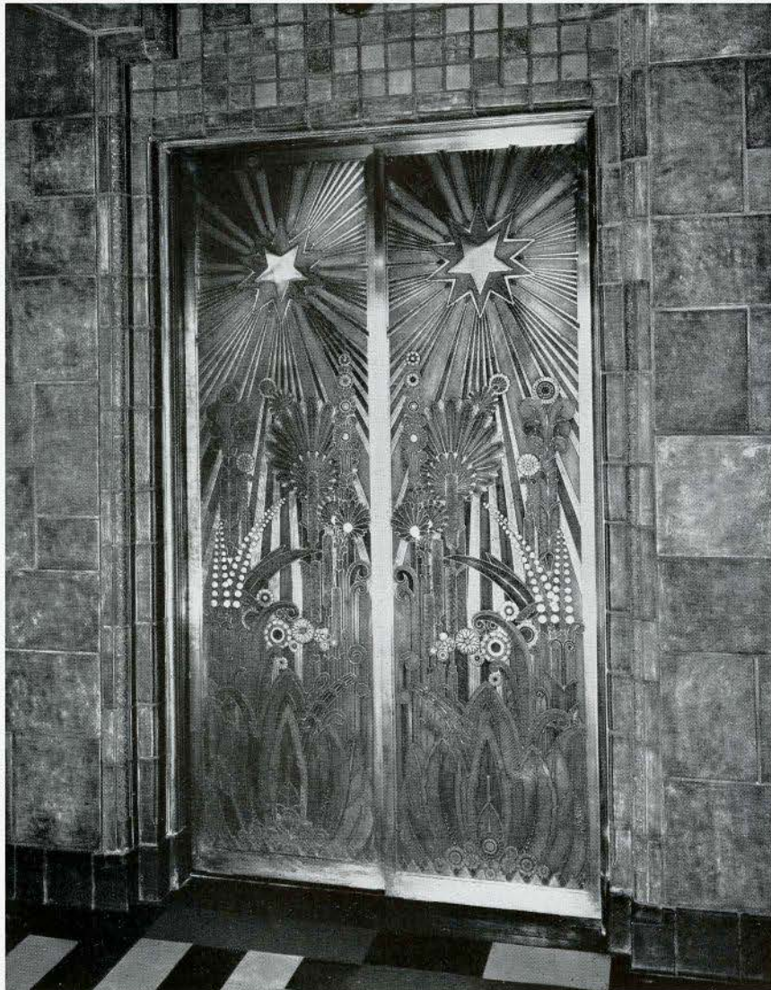
DETAIL OF ELEVATOR DOORS THE MARINE BUILDING, VANCOUVER, B.C.
