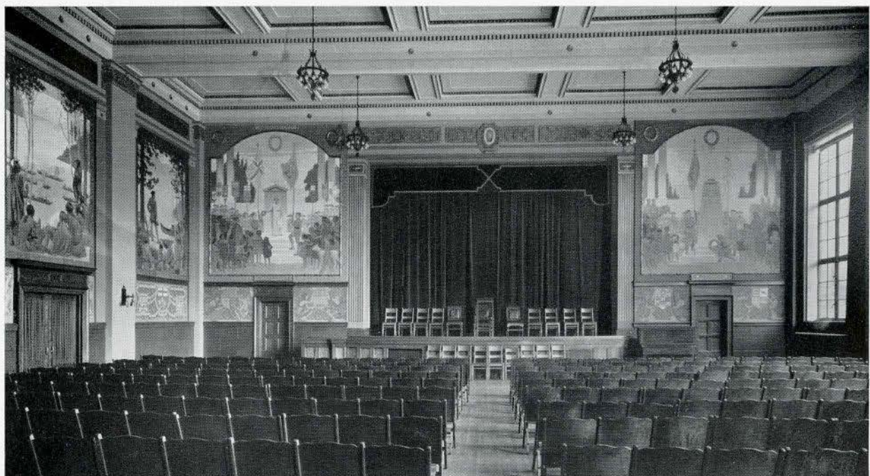
GENERAL VIEW OF AUDITORIUM
