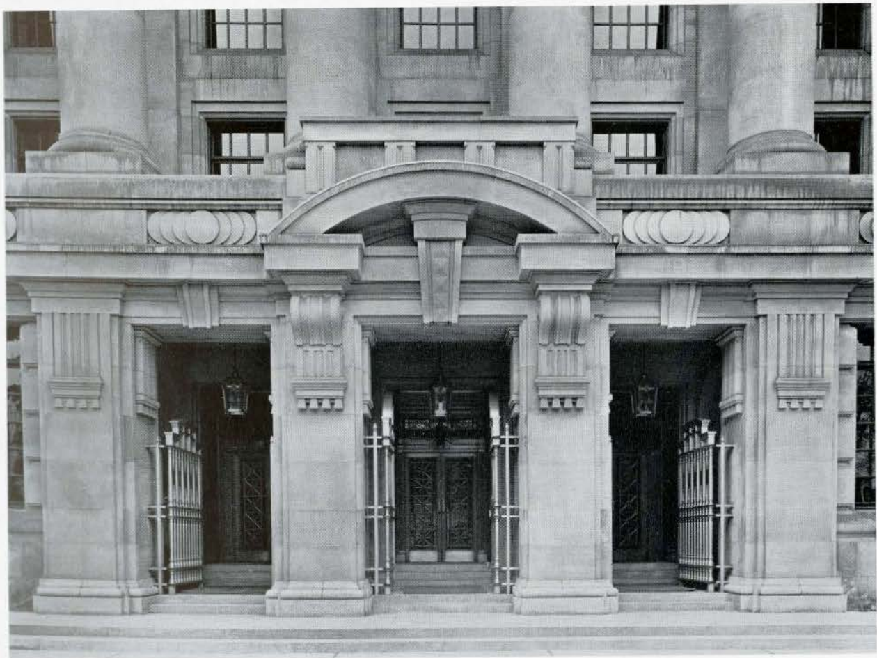
DETAIL OF MAIN ENTRANCE
