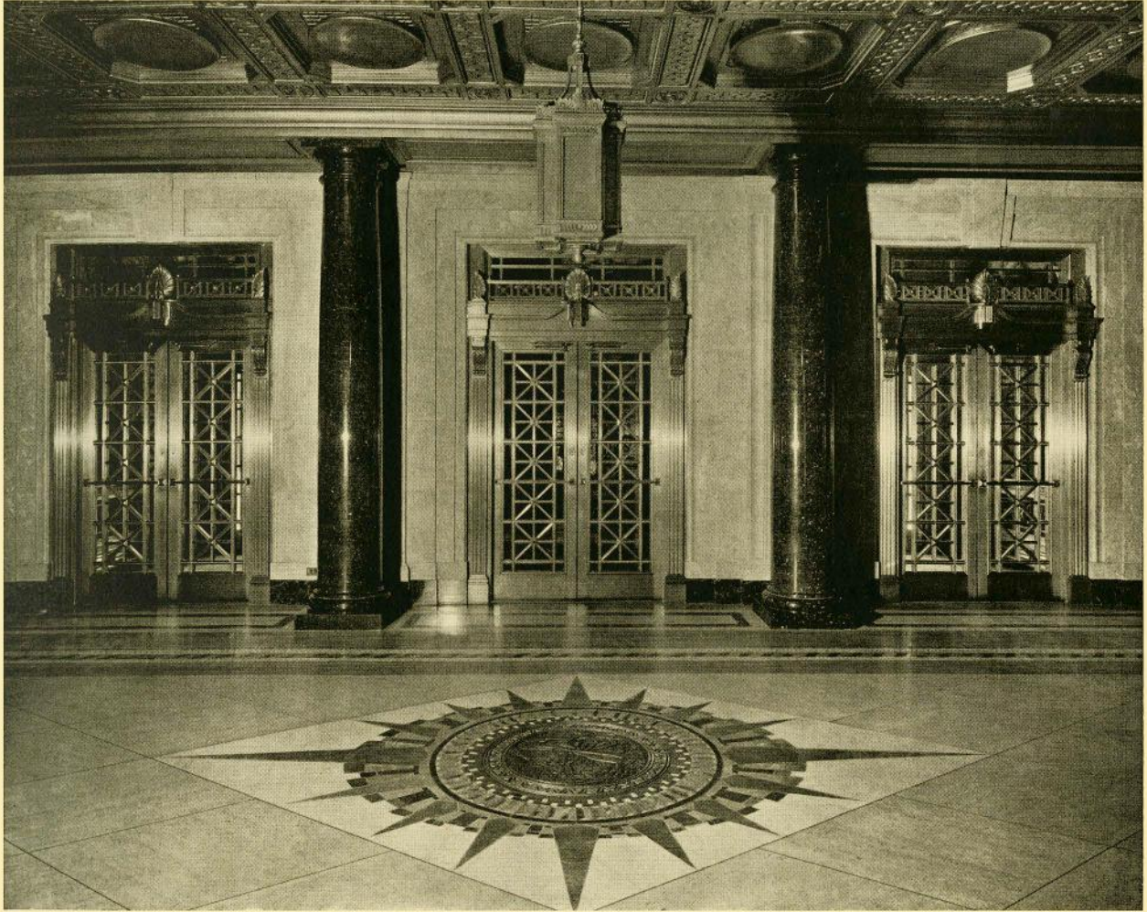
DETAIL OF ENTRANCE HALL CANADA LIFE BUILDING, TORONTO Sproatt & Rolph, Architects
