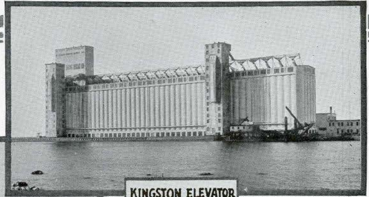
KINGSTON ELEVATOR KINGSTON ONT.
