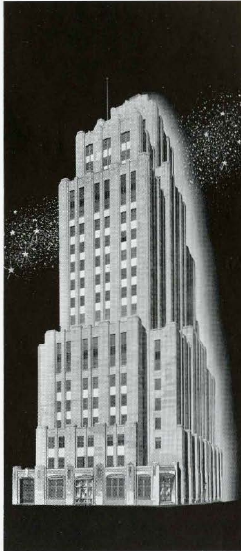
The Aldred Building Montreal
