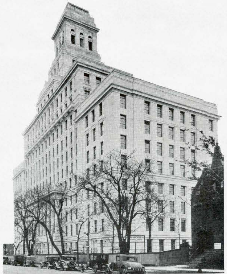
New Head Office Building Canada Life Assurance Co., Toronto
