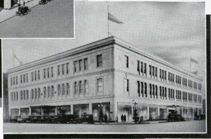
The T. Eaton Co. Building, Saskatoon Architects: Ross and Macdonald, Montreal. Associate Architect: F. P. Martin, Saskatoon. Heating Contractor: Sheppard & Abbott, Toronto. (Photo below.)
