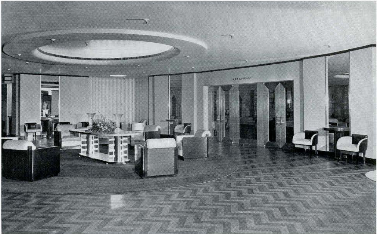
Parquetry Floor of Walnut and Oak in Herringbone pattern, supplied and installed by
