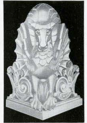
Detail—Corner ornaments at 8th floor level
