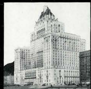
Royal York Hotel—Toronto Ross & MacDonald—Sproatt & Rolph, Associate Architects
