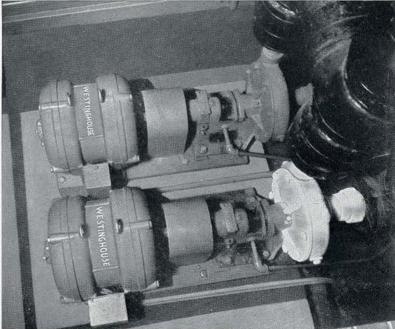
View from above of Westinghouse motors driving De Laval Brine Pump, furnished through Canadian Ice Machine Company. (Above)
