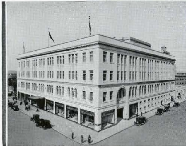
The T. Eaton Co. Building, Calgary Architects: Ross and Macdonald, Montreal. Consulting Engineer: Walter Armstrong, Montreal. Heating Contractor: Pike Bros., Saskatoon. (Photo above.)
