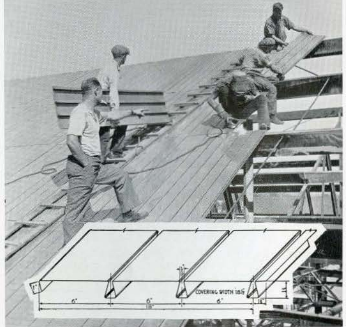
Can. General Electric Building No. 16, Peterborough Contractor: T. A. Brown Company, Limited
