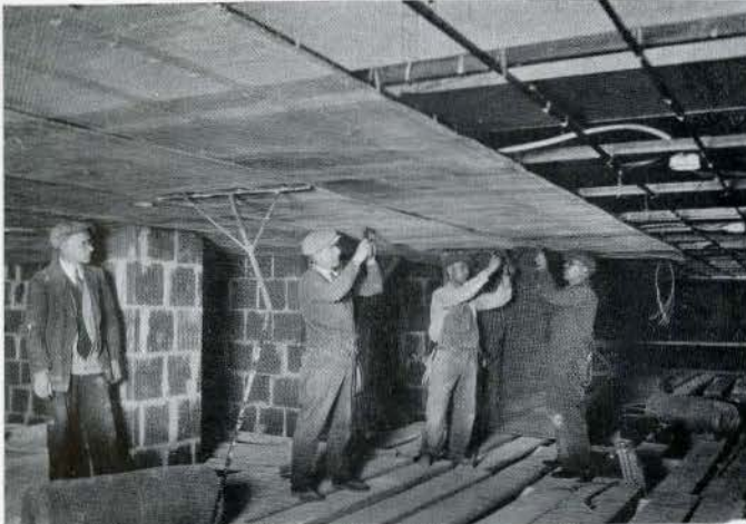
View showing construction of lath on suspended ceiling.
