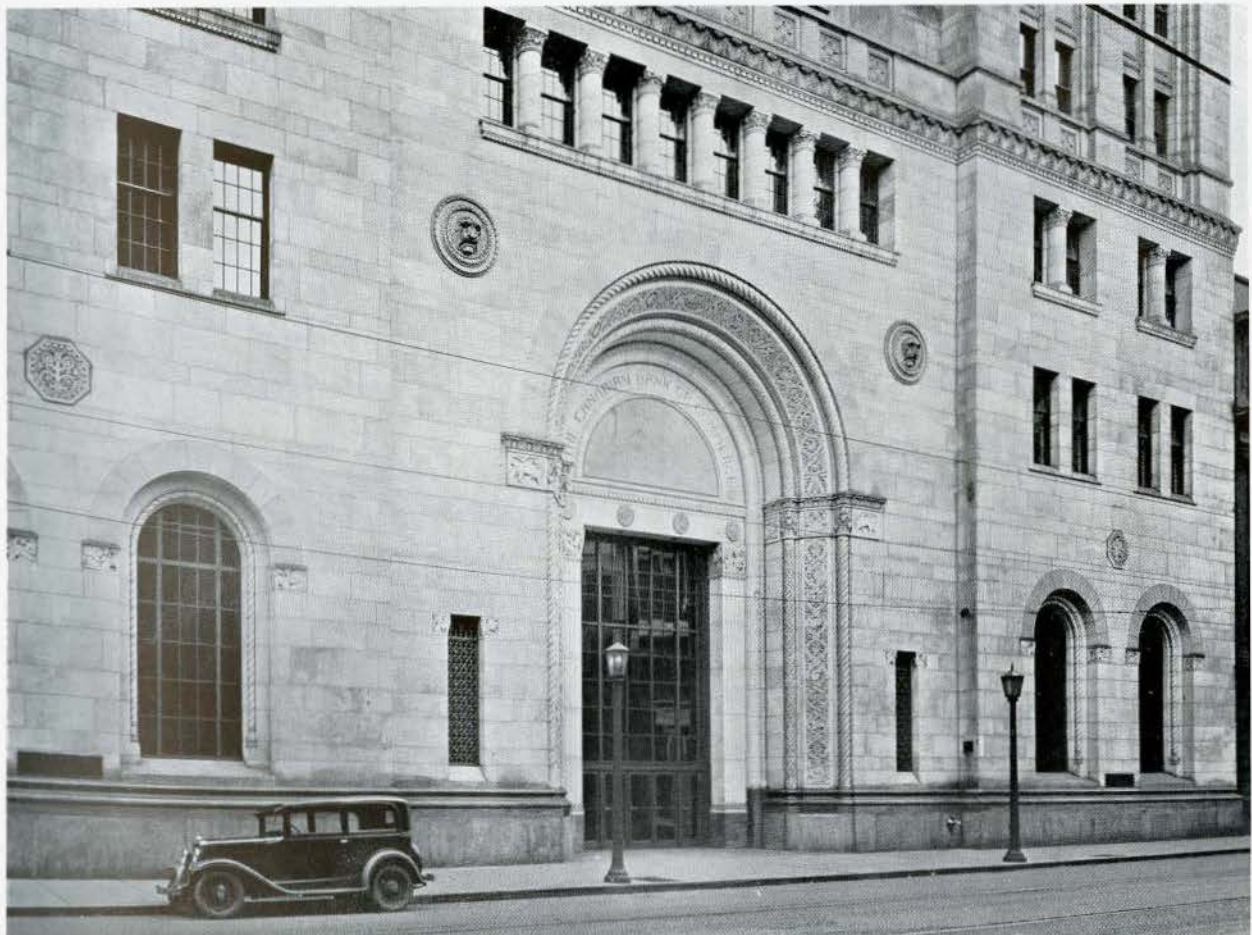
DETAIL OF MAIN FACADE
