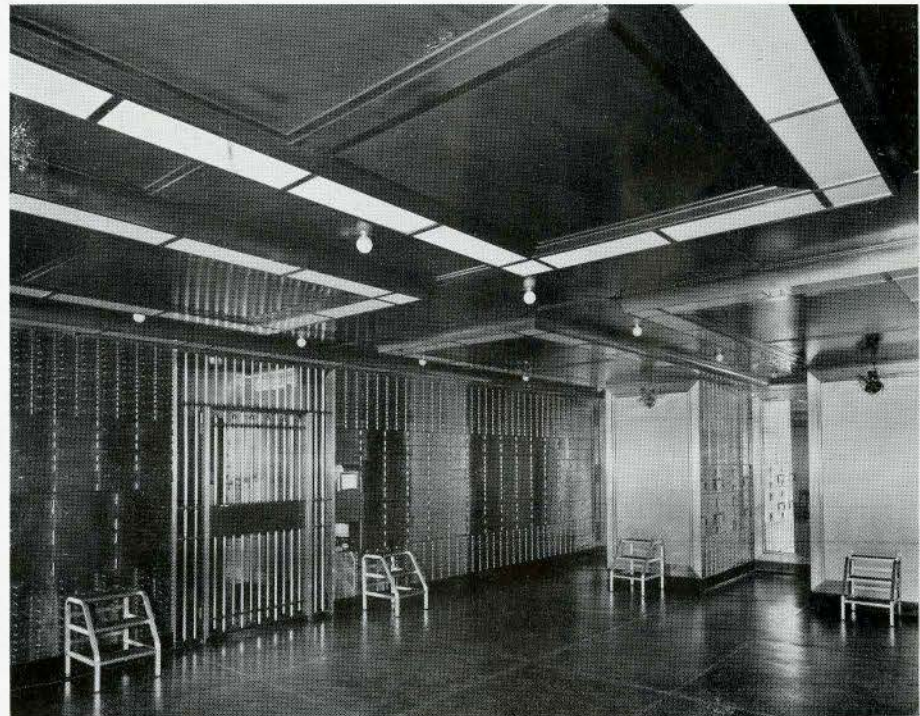
Centre—View showing interior of safety deposit vault in which we installed 3500 safety deposit boxes of Monel Metal.
