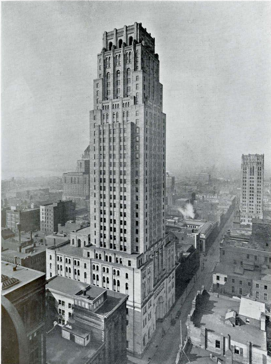
CANADIAN BANK OF COMMERCE BUILDING, TORONTO Darling & Pearson, Architects York & Sawyer, Consulting Architects
