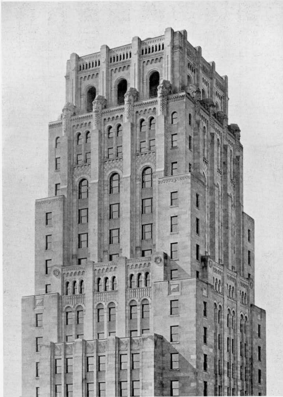
DETAIL OF UPPER STOREYS
