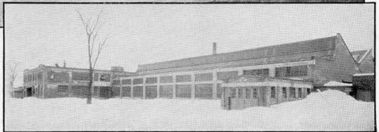
Above—General view of the new Mitchell Foundry.
