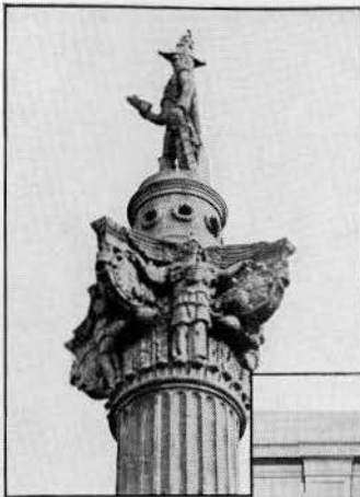
Top of Brock's Monument. Details perfect after seventy-five years. Constructed of Queenston Limestone.
